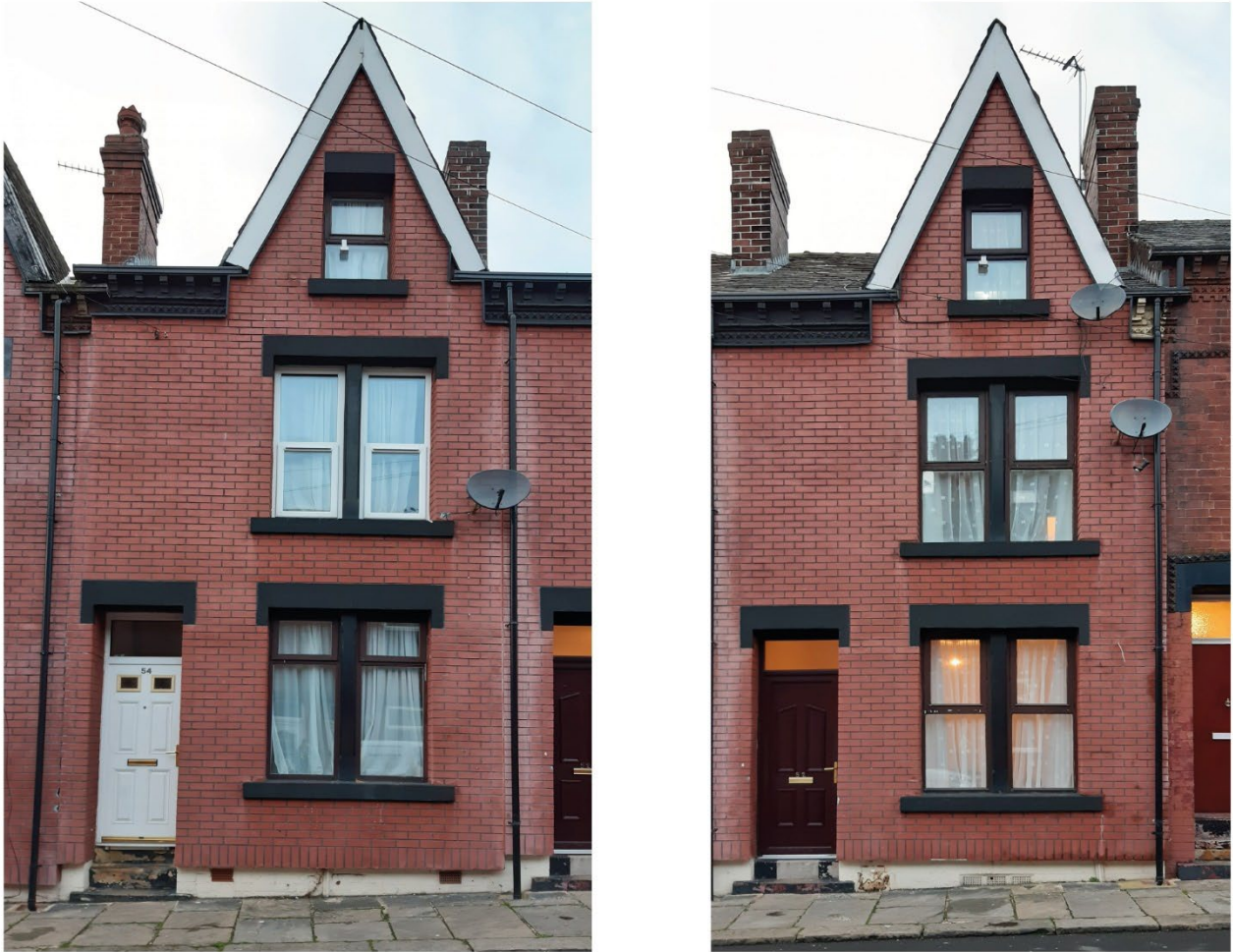
Figure 1-1 Case study houses 54NP (left) and 52NP (right)
