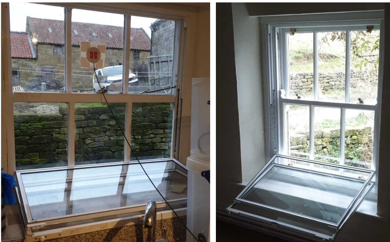
Figure 1-6 Secondary glazing removed for final test phase
