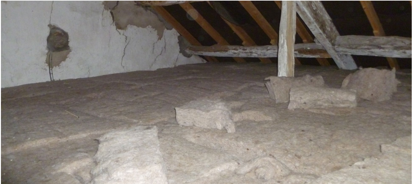
Figure 3-8 200 mm sheep's wool loft insulation – view from loft hatch
