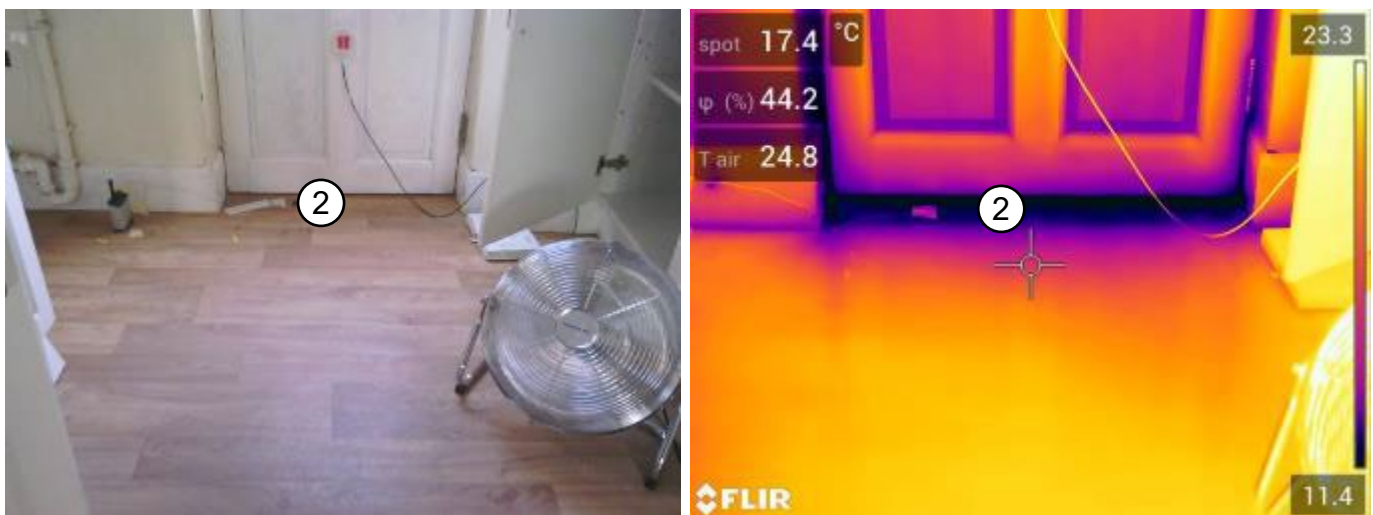
Figure 3-61: Rear door threshold (2) thermocouple sensor location.
