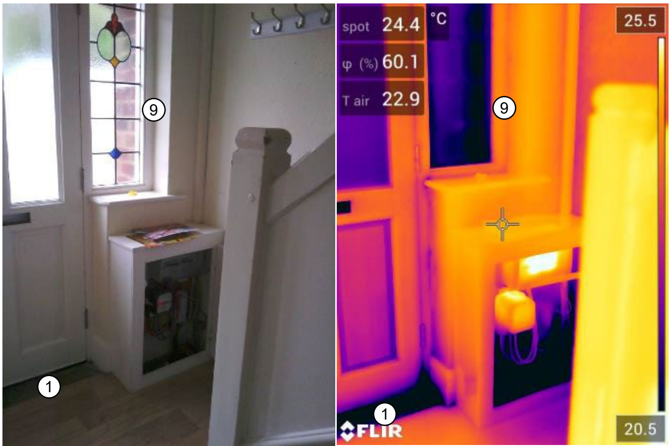
Figure 3-60: Front door threshold (1) and Door opening (9) thermocouple sensor locations.
