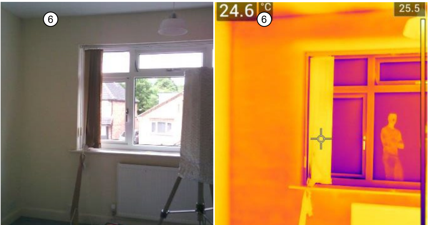
Figure 3-65: External wall to eaves (6) thermocouple sensor location
