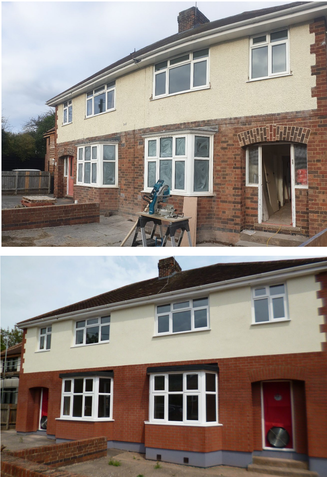
Figure 3-25 55AD & 57AD pre- (top) and post- (bottom) retrofit
