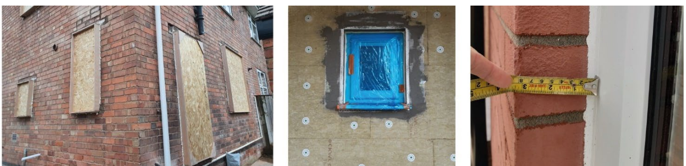
Figure 1-6 Windows and doors installed within plywood box and EWI (55AD)
