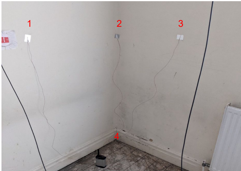
Figure 3-35 Bedroom 1 - front wall to party wall junction, surface temperature sensors.
