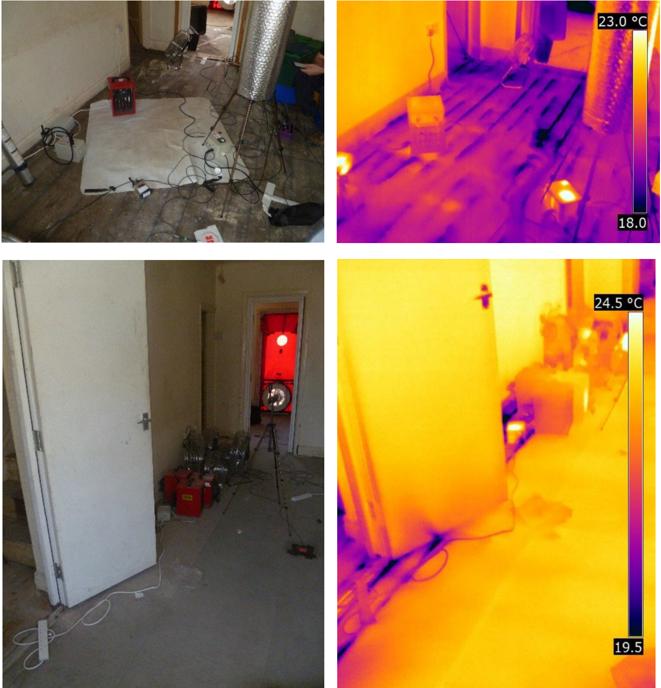
Figure 3-2 Air leakage through the suspended ground floor was reduced with the replacement floor covering
