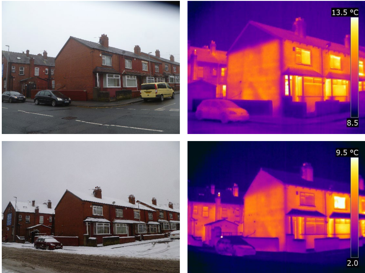
Figure 3-16 Comparison of old windows and doors (top) and replacements (bottom) on the front façade during coheating phases
