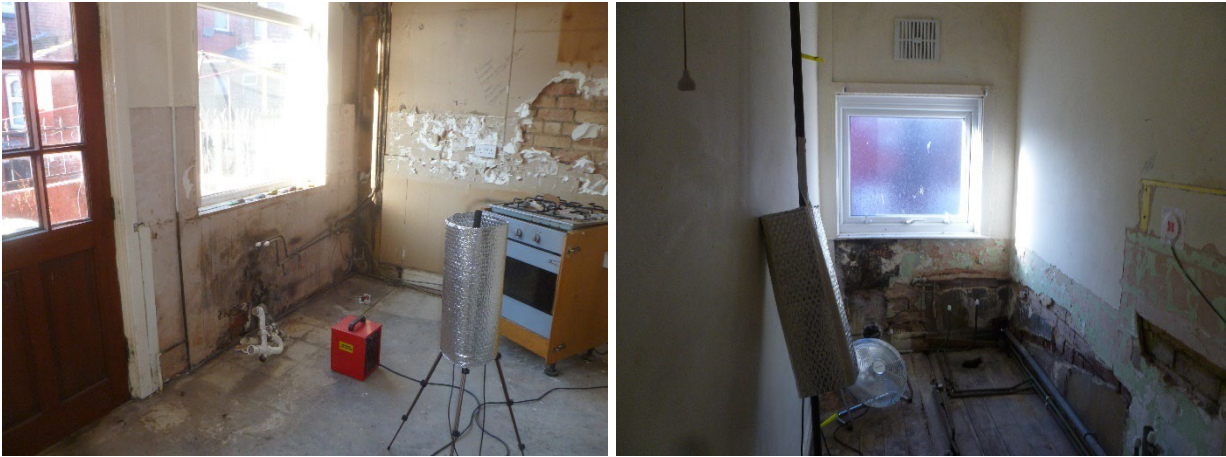
Figure 1-5 Kitchen and bathroom with fittings removed prior to testing
