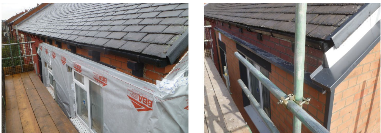
Figure 3-20 EWI was installed up to the underside of the corbels, where an insulated render based EWI system was used to accommodate the brickwork feature.
