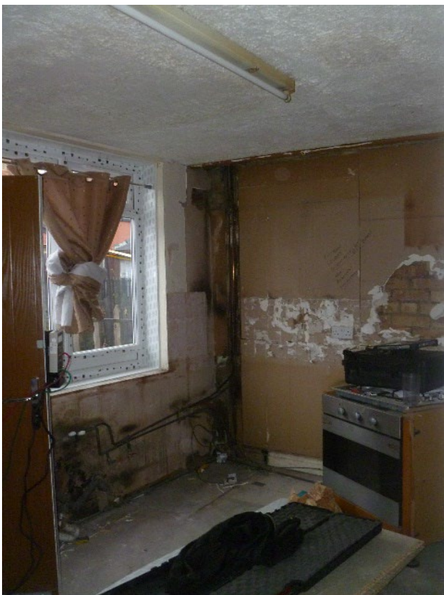
Figure 3-3 Infiltration in the kitchen into the void behind the dry lining under depressurisation observed at Stage 3 of the retrofit (01BA.R.G)
