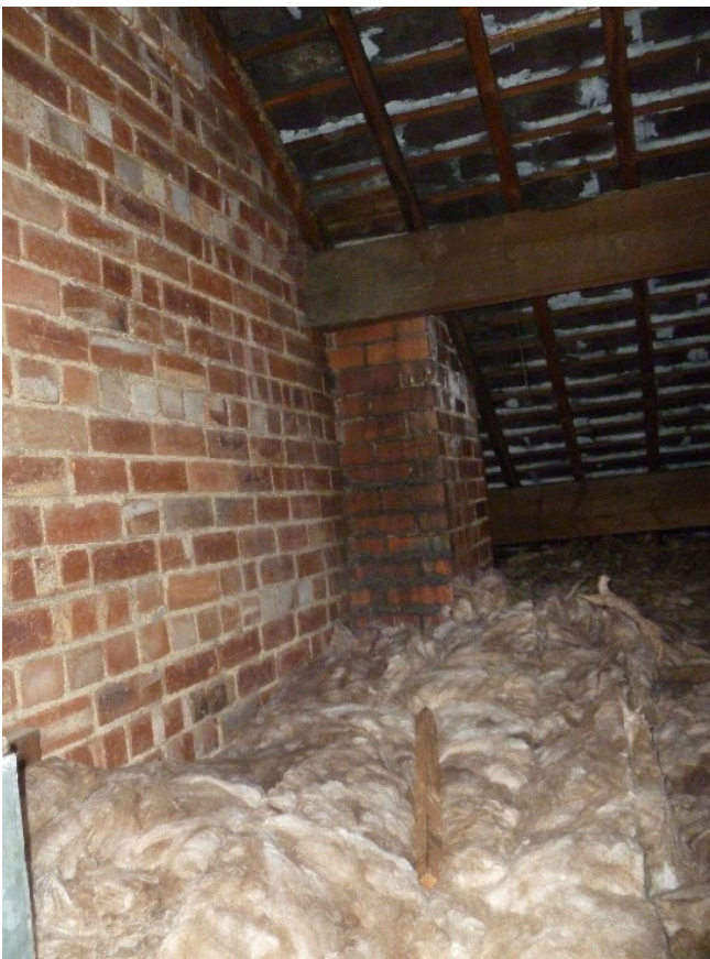
Figure 3-15 Comparison of original loft insulation (top) and new (bottom) showing bypassing and bridging at the chimney breast and the intersection between the party wall and the first-floor ceiling.
