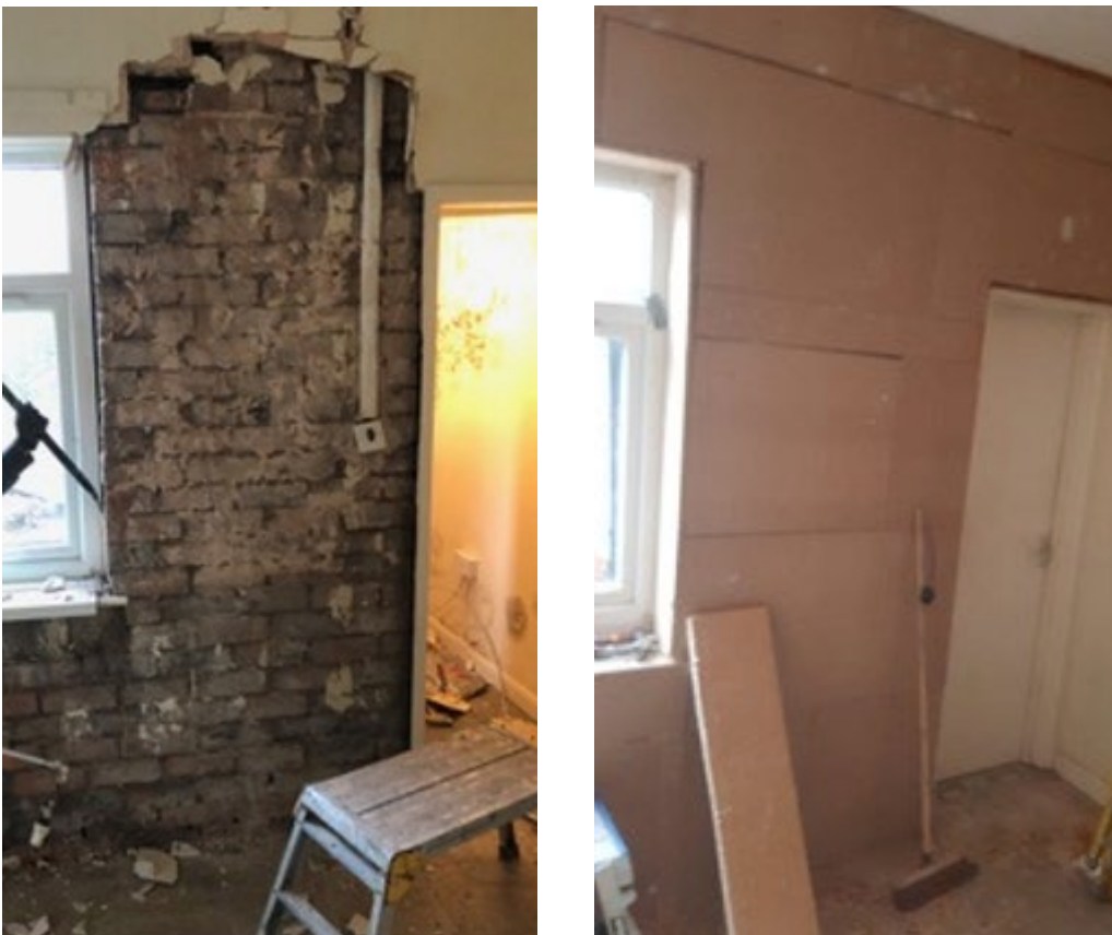
Figure 3-15 Wood fibre IWI being fitted on the front and rear wall
