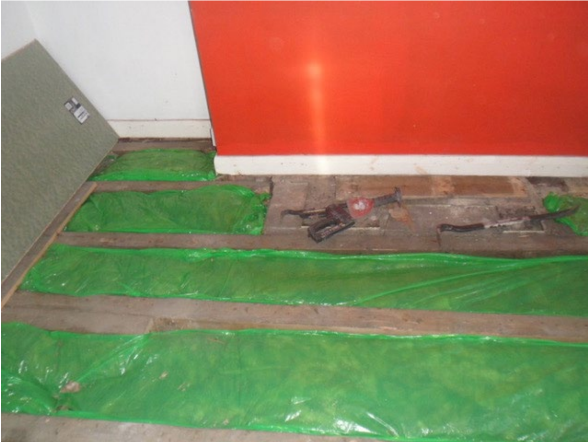
Figure 3-13 Suspended floor insulation
