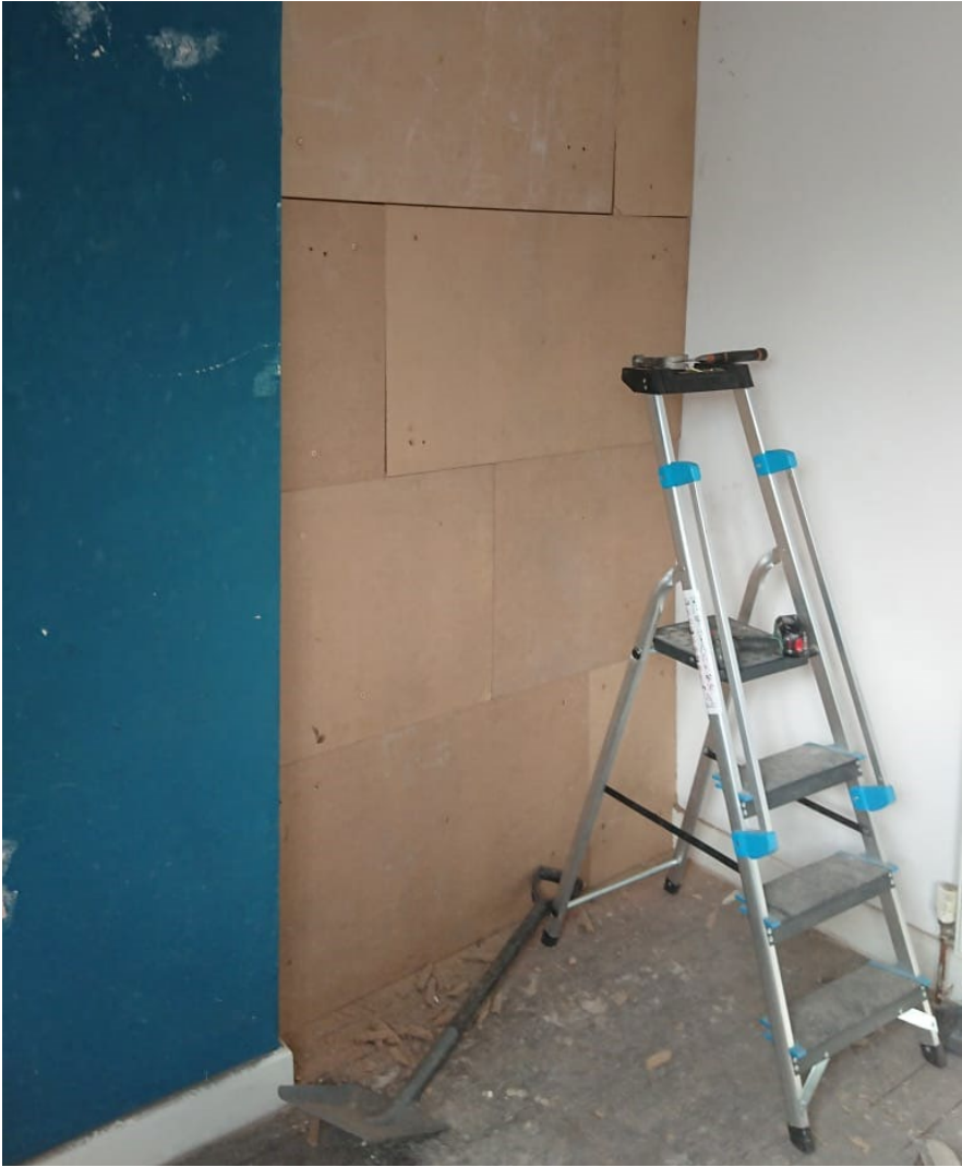
Figure 3-13 Gable wall insulation mid-retrofit (17BG.A.R)
