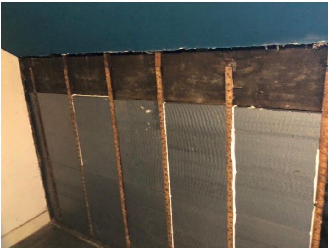
Figure 3-12 Knee wall insulation mid-retrofit (17BG.A.R)
