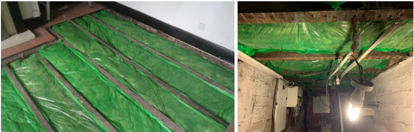
Figure 3-15 Suspended timber ground floor insulation mid-retrofit (17BG.A.R.F)
