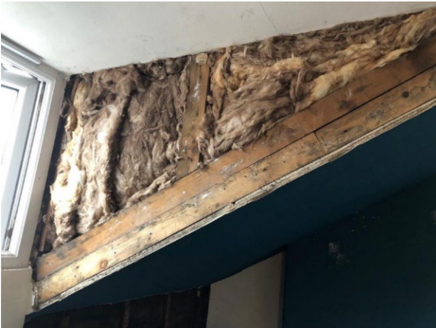
Figure 3-14 Dormer cheek insulation mid-retrofit (17BG.A.R)
