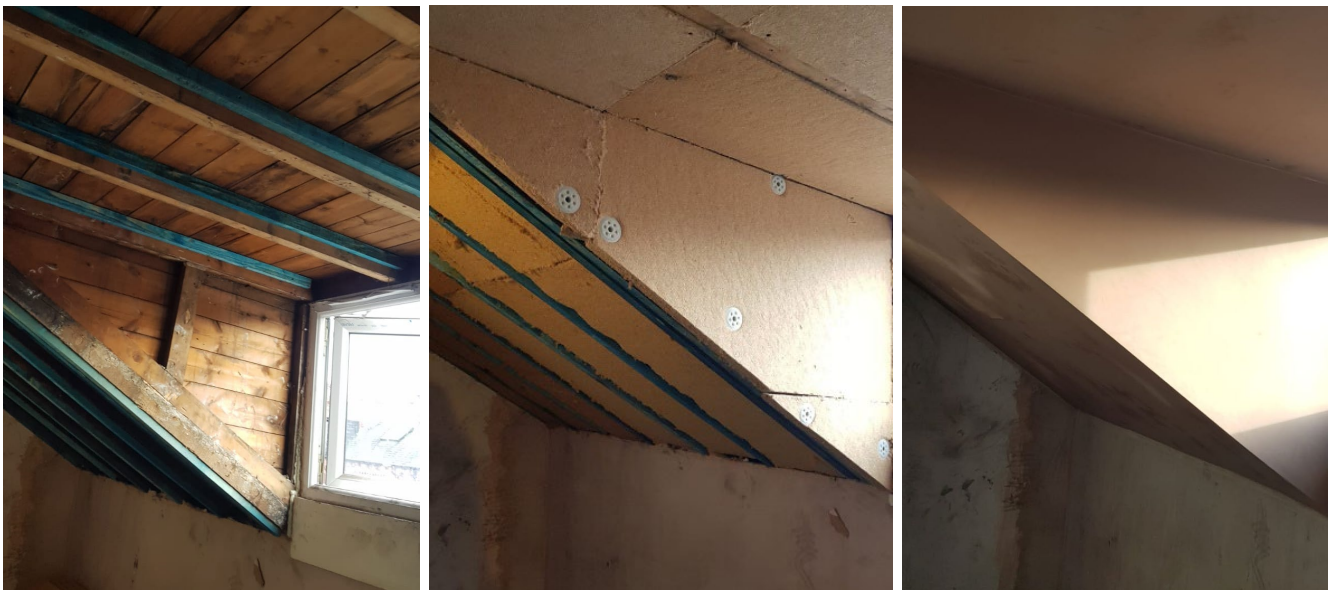
Figure 3-19 Dormer roof, cheeks and sloping ceiling insulation retrofit stages (17BG.A.R.F.W.WH)
