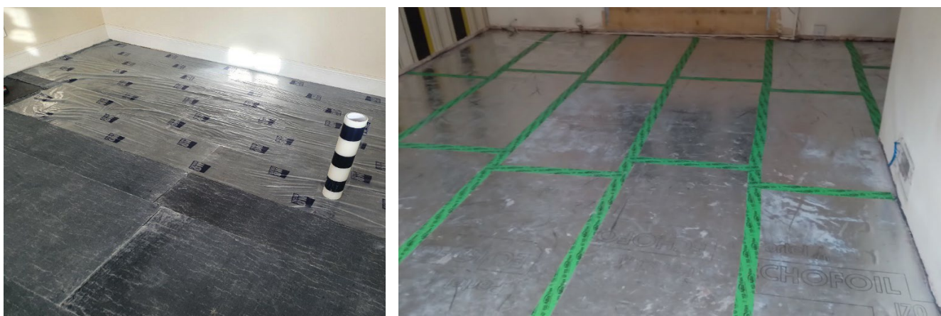
Figure 1-18 Left: 10mm aerogel blanket, Right: 20mm aerogel panel
