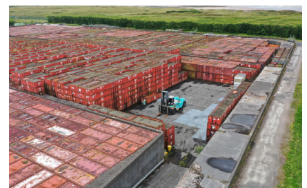
The 'tennis court' area in Vault 8 is ready and waiting to receive its final waste containers
