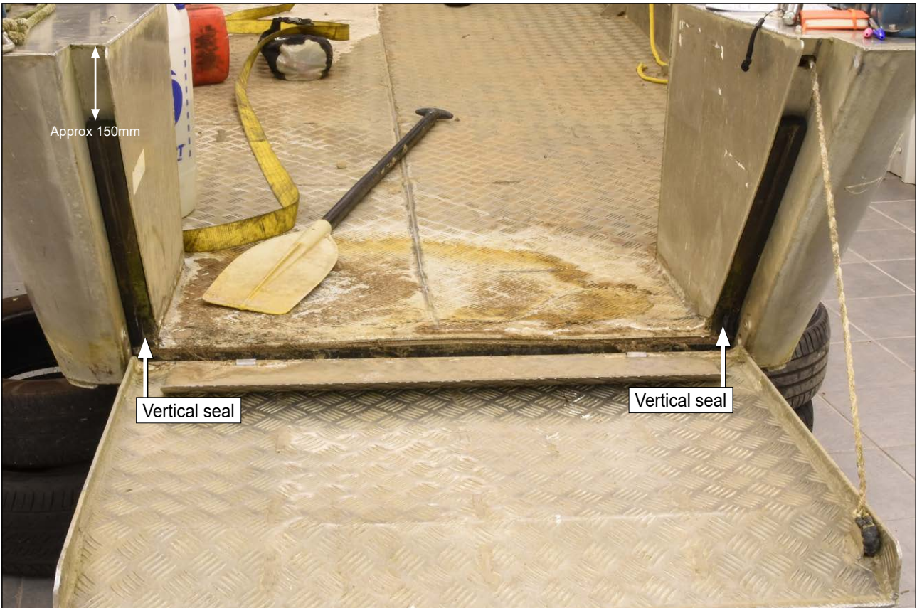
Figure 13: Bow ramp vertical seals 150mm lower than the top of the ramp
