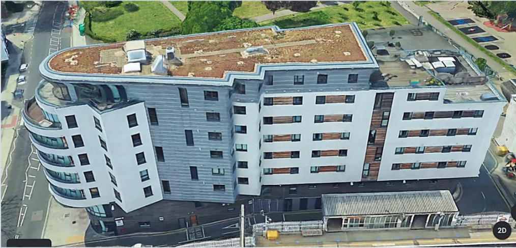
East Façade: Elevation D
