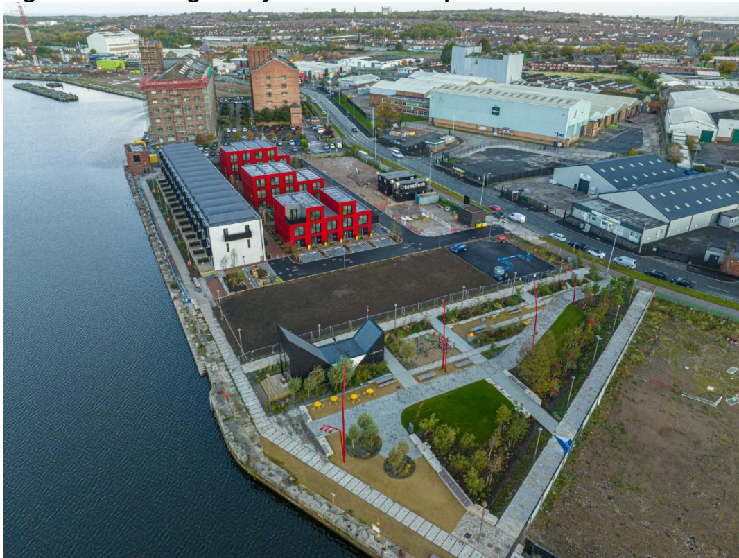
Figure 6: Redbridge Quay modular development
