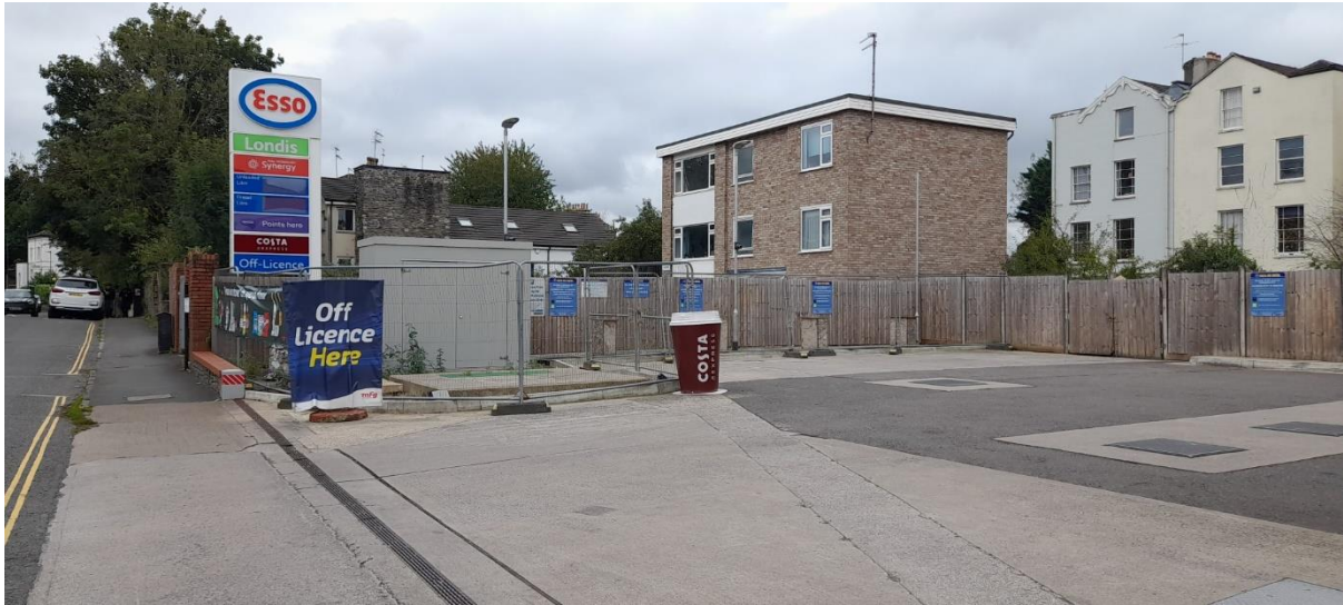
The substation and charging points. Not conspicuous compared to huge Esso sign, advertising banners, Costa Coffee cup, flat roofed apartments and boundary fence.
