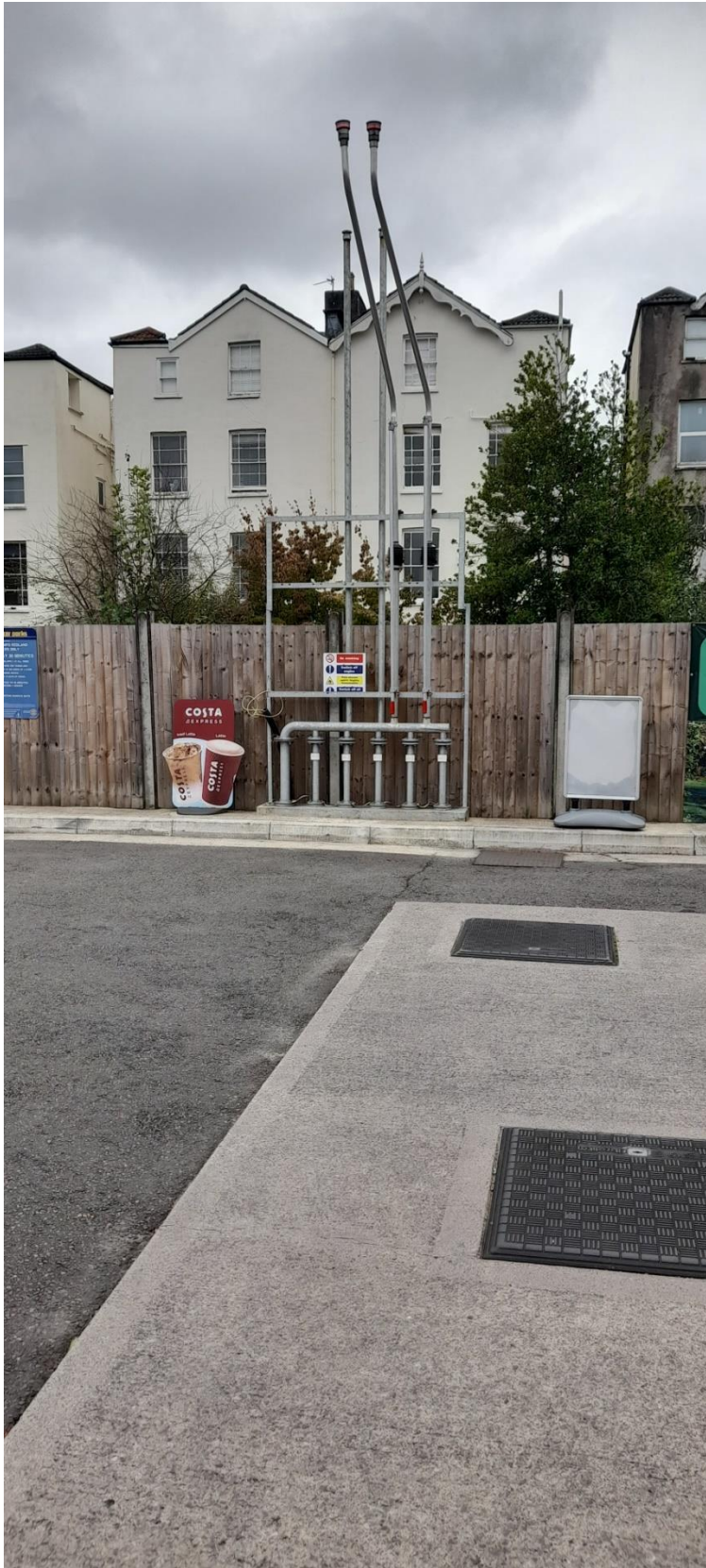
View of Pipe Assemblage. No conservation value here.
