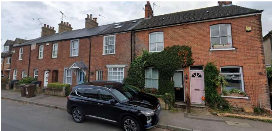
View of the nearby terraces at no.4 to 14 St.Annes Road
