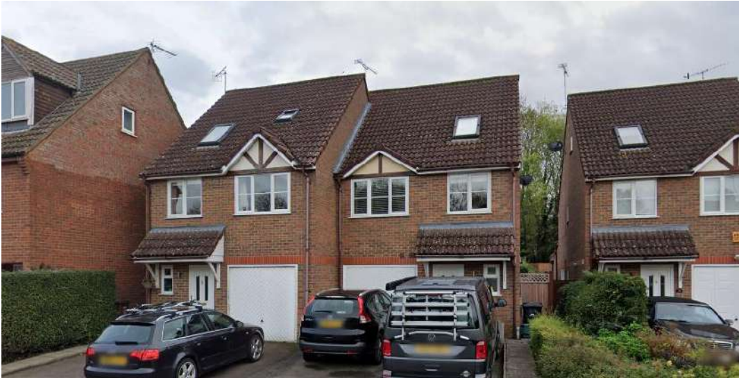
Relationship between existing neighbouring dwelling with narrow gaps and full flanking gable ends
