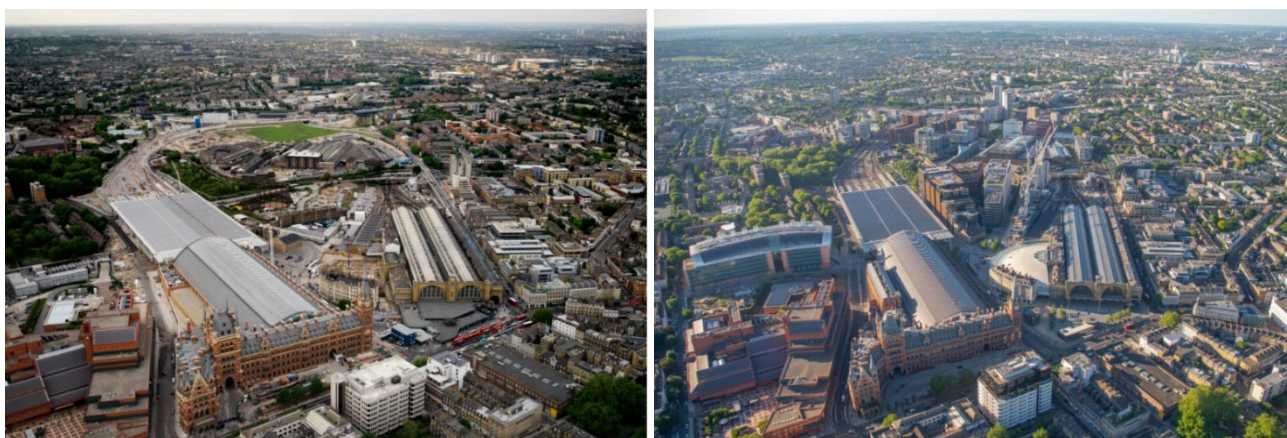
Figure 3.9: St Pancras International and King's Cross stations in 2006 (left) and 2020 (right)
