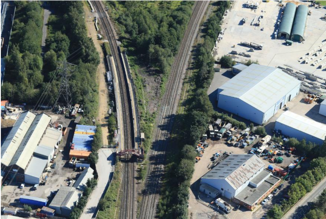
Figure 1 – The existing Ravensthorpe Station is in the left of centre in the picture
