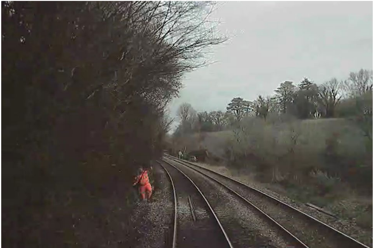
Forward-facing CCTV showing the COSS in the up line cess as the train approaches (courtesy of Great Western Railway).
