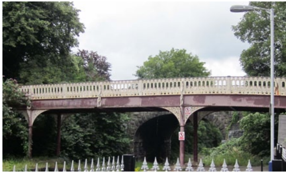
Figure 81: Cast iron footbridge over railway line, from Redland Station
