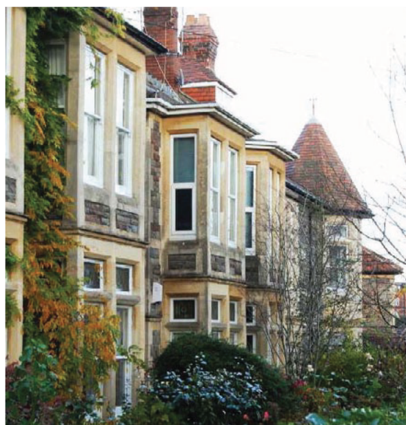
Figure 85: Canarvon Road facades
