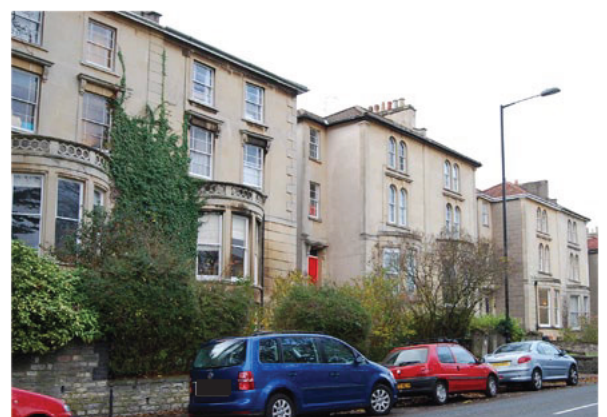
Figure 41: Cotham Grove, 3-storey over semi-basement
