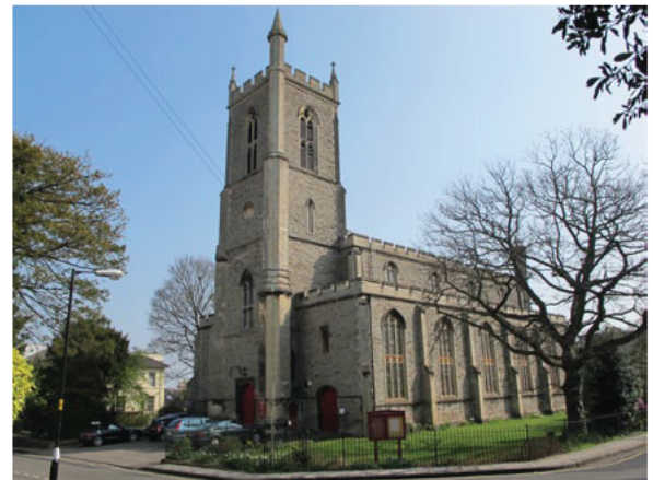
Figure 52: St Matthews Church
