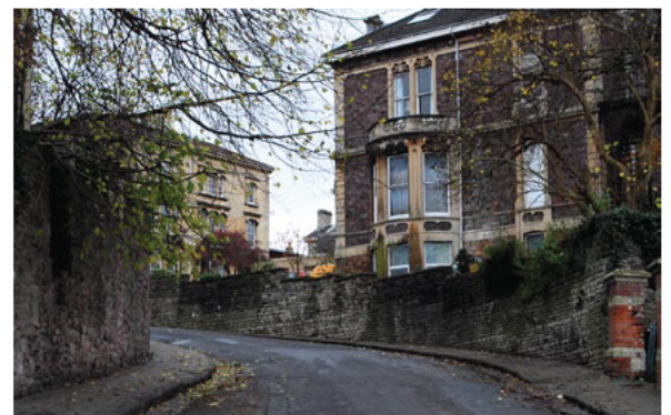
Figure 40: large boundary wall, Archfield Rd
