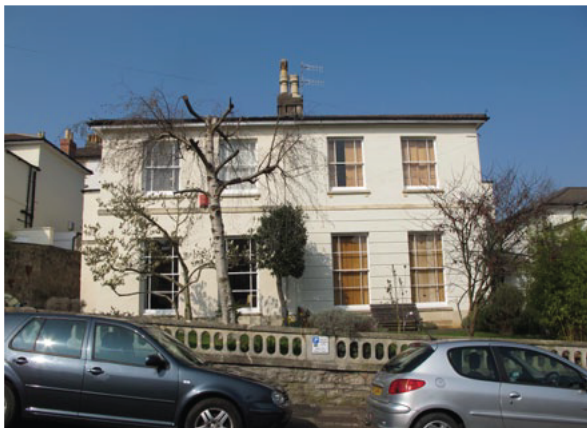
Figure 51: Typical Victorian semi, Clare Road
