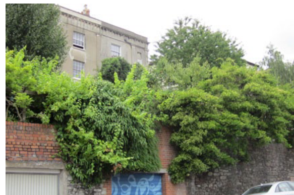
Figure 49: Rear of Springfield Road properties from Sydenham Road
