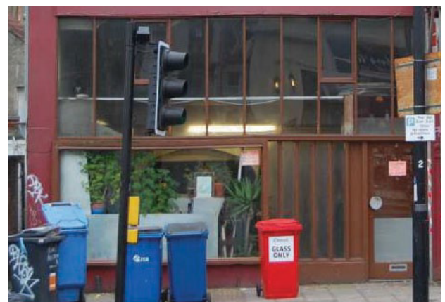
Figure 114: Poor quality shopfront
