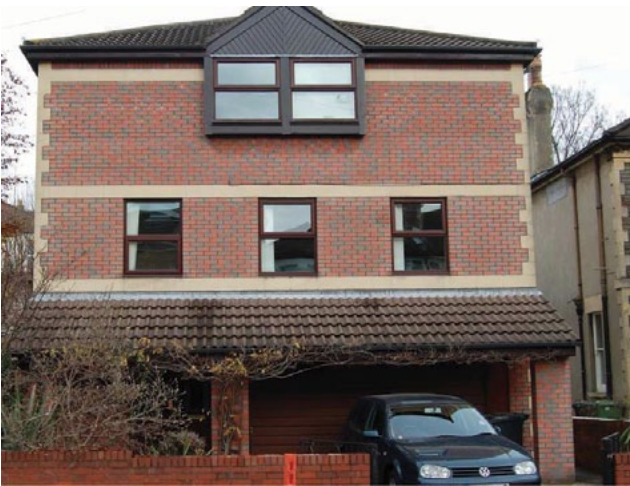
Figure 115: Poorly designed infill
