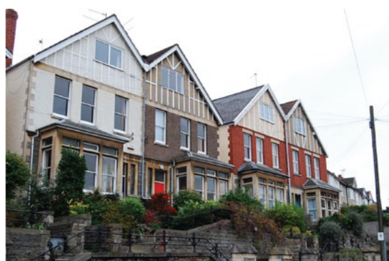
Figure 33: nos. 48 - 52 Trelawney Road
