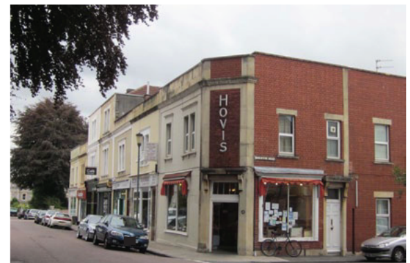
Figure 57: Nos. 1 - 30 Chandos Road
