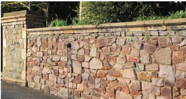
Figure 100: Brandon Hill stone retaining wall, Woodstock Road
