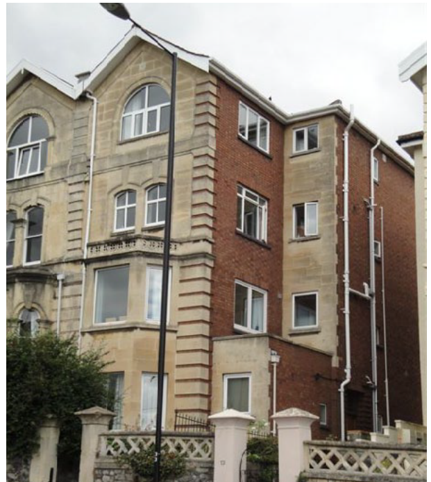
Figure 118: uPVC windows, Redland Road
