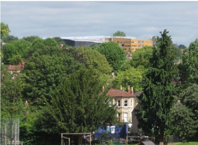
Figure 116: Redland Green School has a negative impact when viewed from the south
