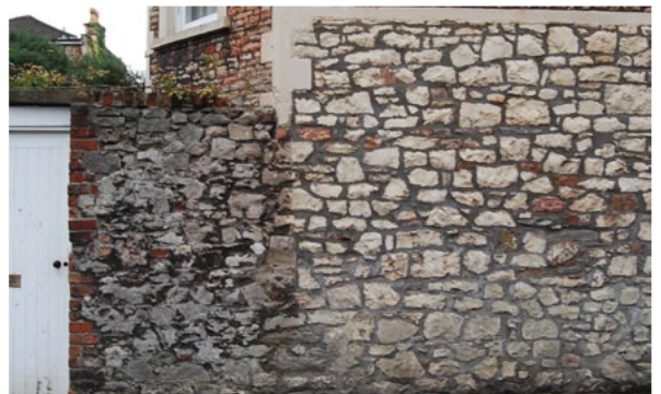
Figure 32: Stone walling materials, Kenilworth Road
