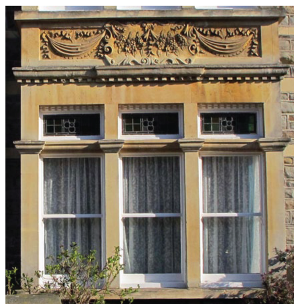
Figure 93: Late Victorian windows, Luccombe Hill
