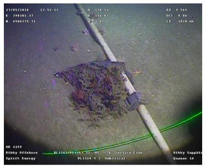
Figure 3-3: Example of fishing debris.
