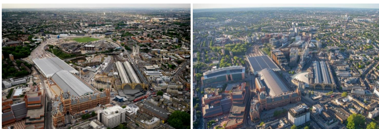
Figure 3.9: St Pancras International and King's Cross stations in 2006 (left) and 2020 (right)
