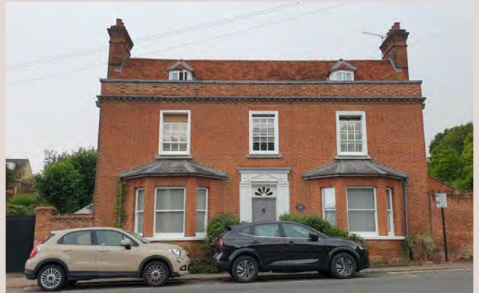
▲ Brewery House adds ornate character to the street through dentil detail and bay windows.
