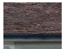
Peg tiled roof
