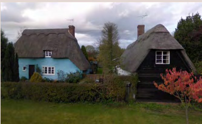
▲ Thatched cottages with contrasting pastel facades in Duddenhoe End adding character to the hamlet.
