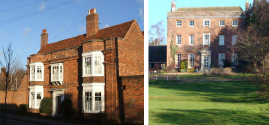
▲ Castle Street, Saffron Walden (left image) and Walden Place (right image) are grand examples of the typical mansion houses in Uttlesford.
