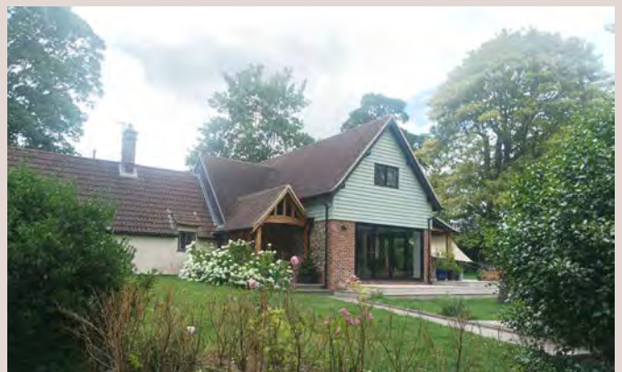
▲ Modern example of house extension in Little Bardfield using local materials such as flint and white weatherboarding.
