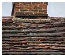
Peg tiled roof
