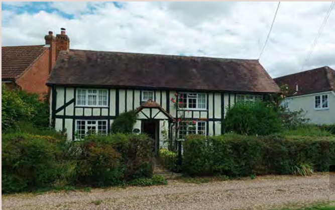
▲ Timber framed cottage with peg tiled roof overlooking Bannister Green. Low hedged boundary treatment integrated with informal shared space.
