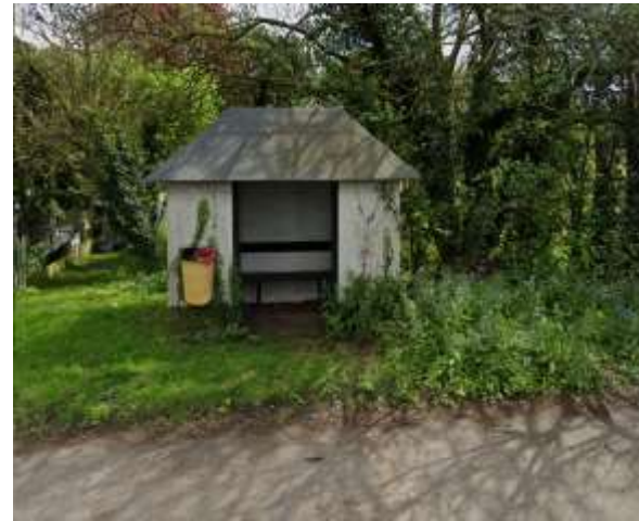
Fig 2. Existing bus stop on B1383 to north west corner of site
