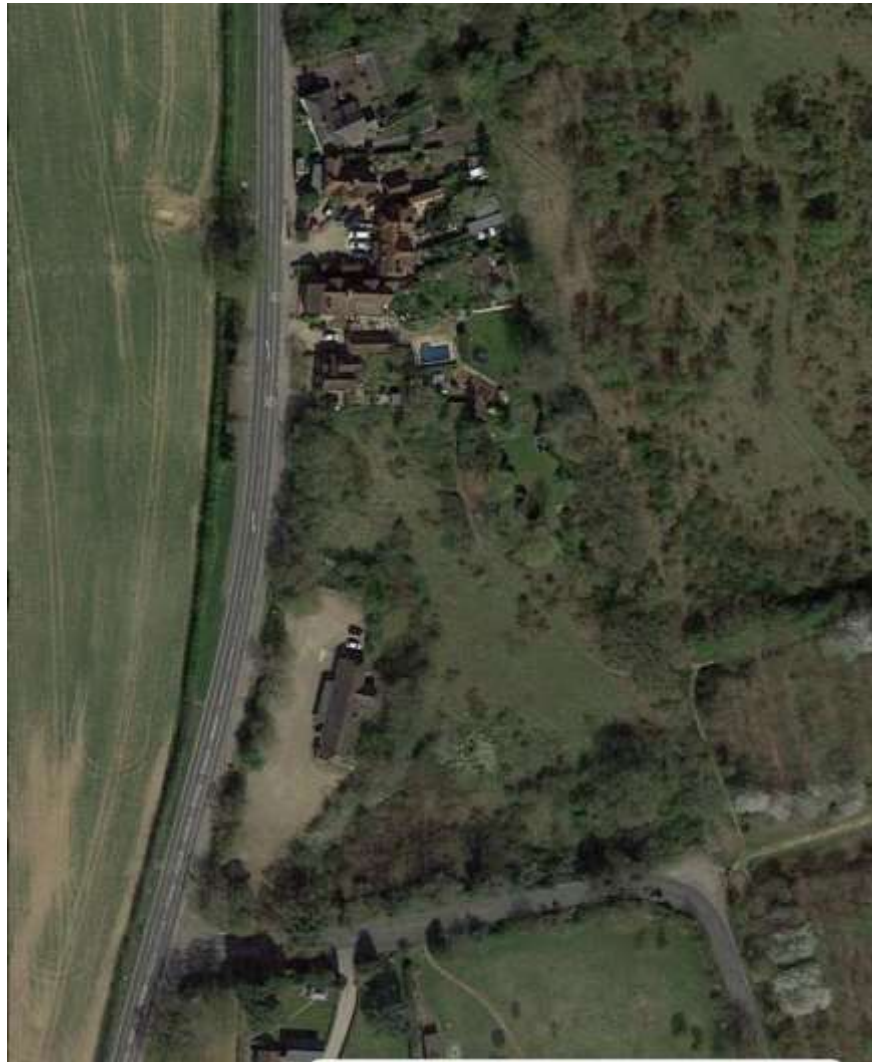
Fig 1. Aerial view of site
