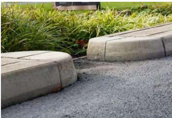
Images of kerb gaps constructed at Beaulieu Park, Chelmsford - Images courtesy of ECC SUDS Design Guide 2020
