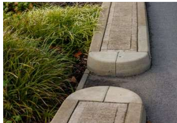
Images of kerb gaps constructed at Beaulieu Park, Chelmsford - Images courtesy of ECC SUDS Design Guide 2020
