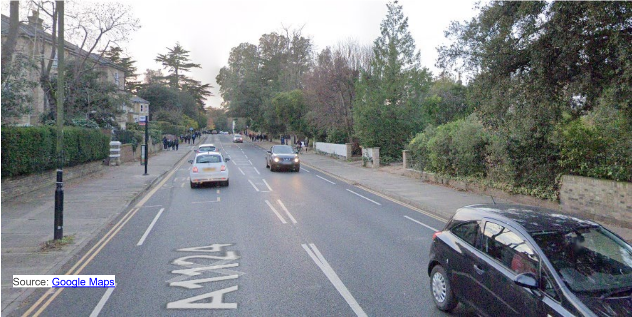
Figure 8 Looking west along the scheme route (Lexden Road) with its current painted cycle lane provision on either side of the road
