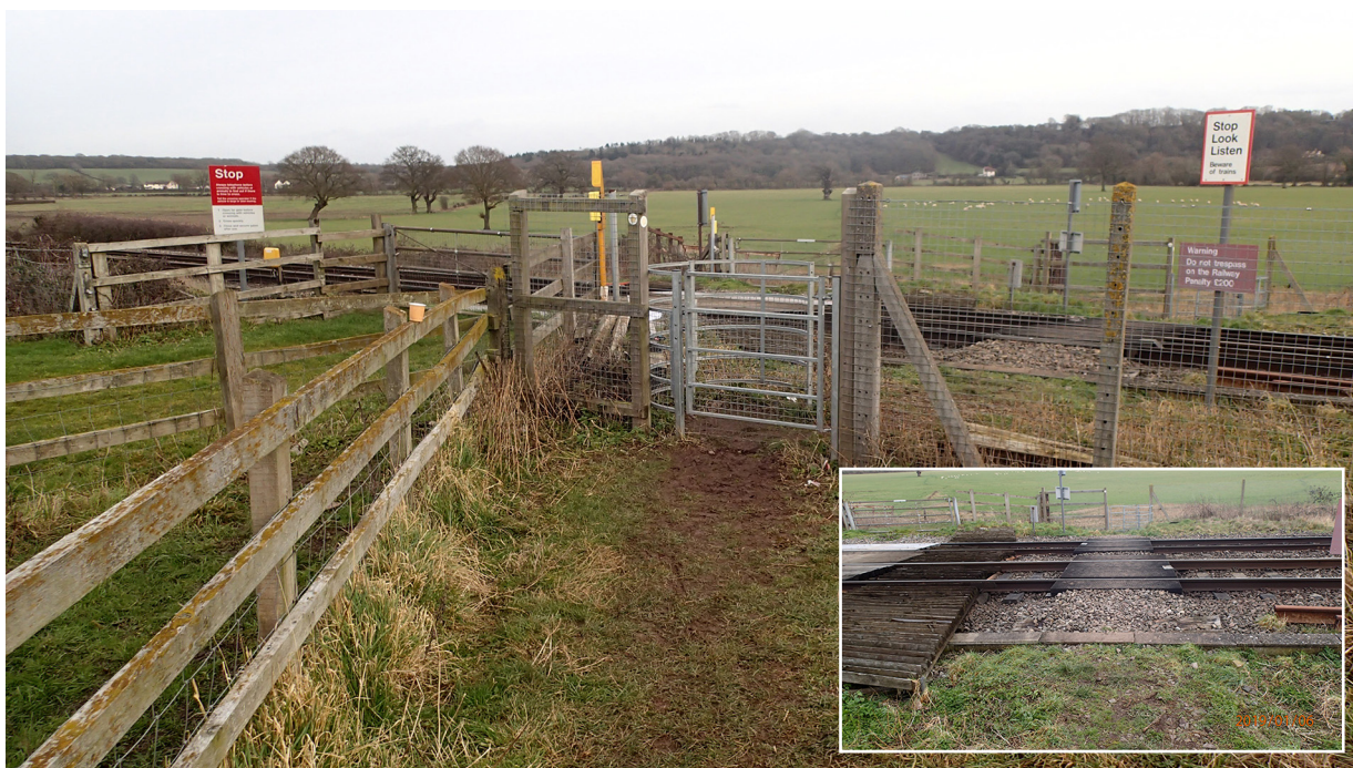
Figure 5: Significant features of Tibberton No. 8 footpath crossing when approaching from the west
