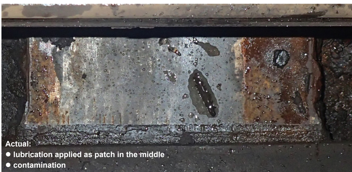
Figure 9 – Switch rail to baseplate interfaces (representative examples)
