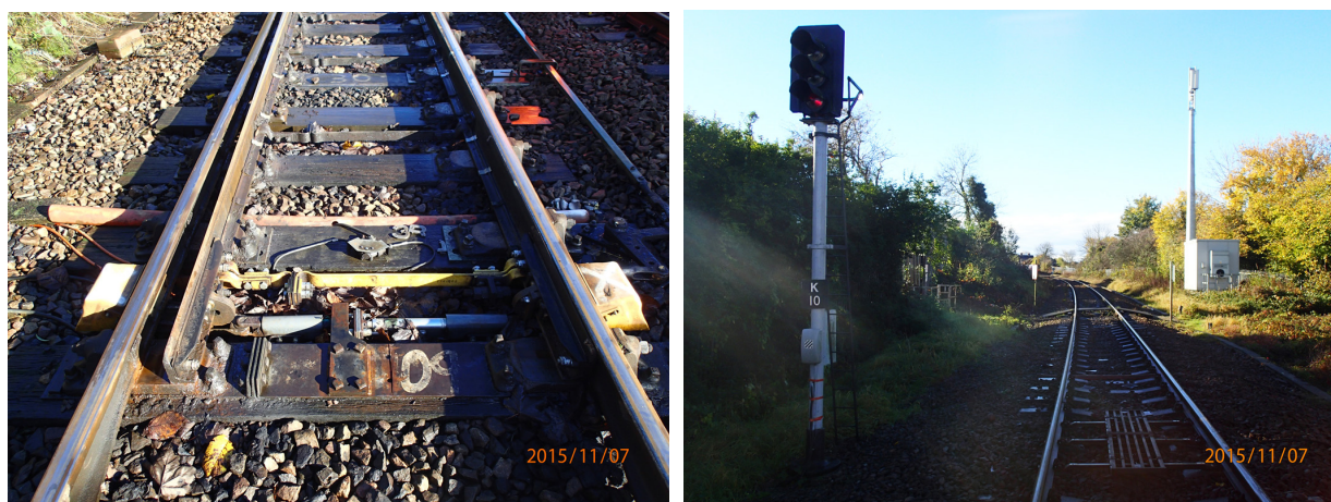
Figure 4: Points 3 in the 'normal' position and signal K10
