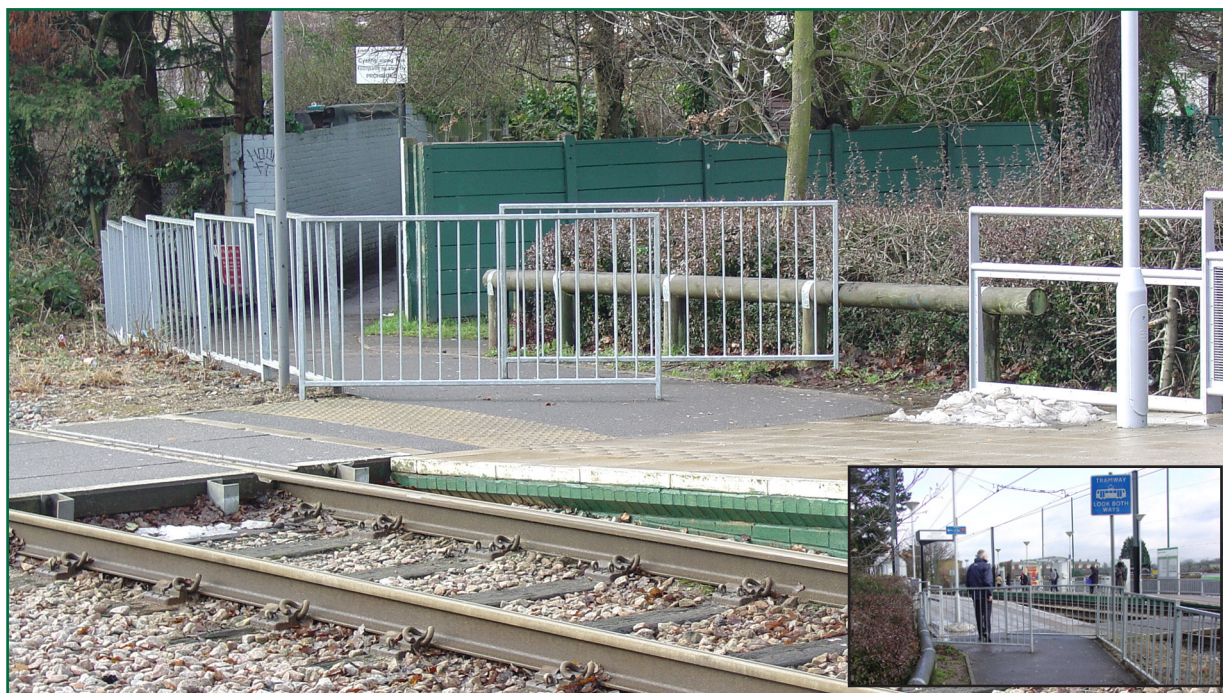
Figure 7: Chicane installed at Arena tram stop
