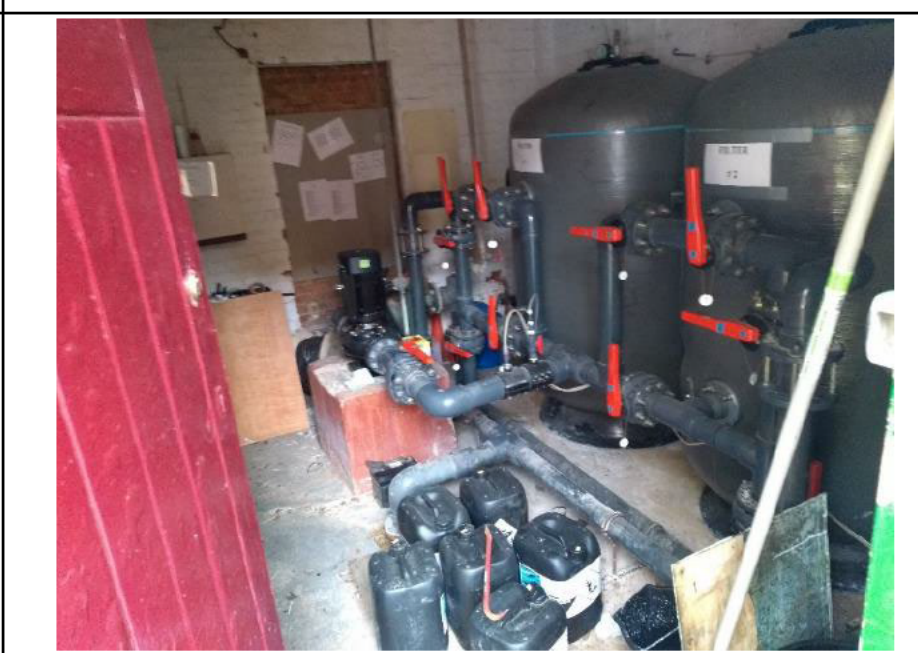
6 - Example of plant room with several containers of adblue stored in foreground
