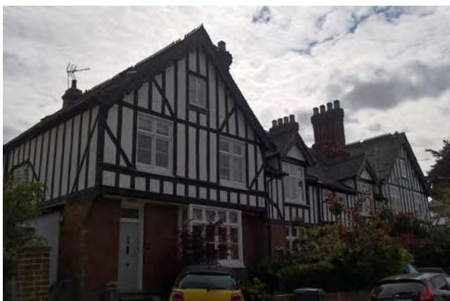
Picture 1.51 No.s 39 - 45 West Road, a terrace of two storey houses dating from the late 19th century with exquisite detailing including pargetting, decorative bargeboards and prominent brick chimney stacks.
