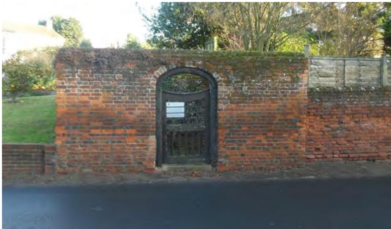
Picture 1.11 The Pound enclosure located on Little Walden Road, with brick elevations in English Bond and an opening with wooden door to the west elevation. There is a further blocked opening on the north elevation.
