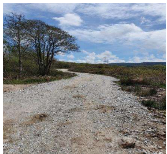
Photo 8. Example of stone resurfacing undertaken at Gothers track - Goss Moor, January 2021
