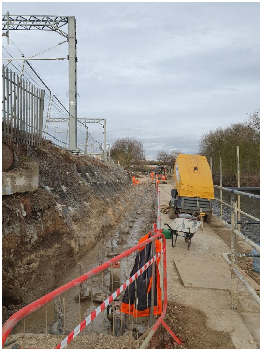
Bank repair on the River Don, Rotherham
