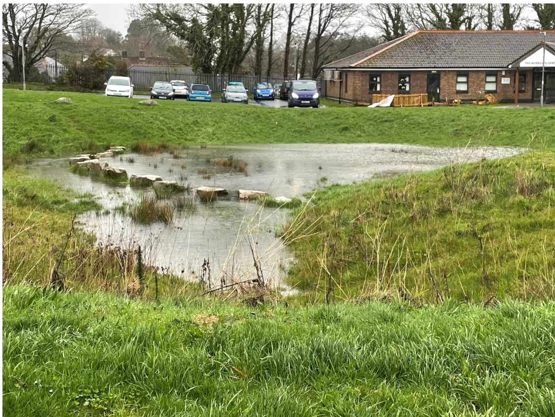
Natural Flood Attenuation measures at Bull Engine Park (Par Lane/Burrows Centre)
