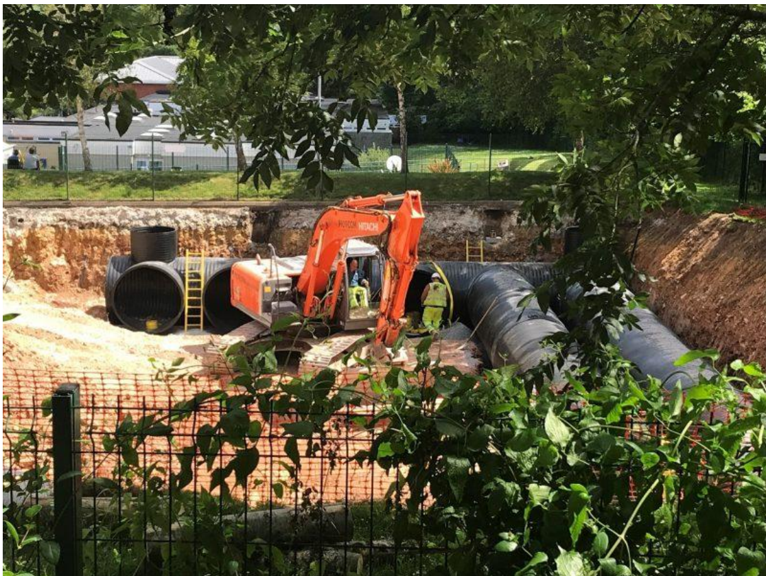
Installation of the Attenuation Tank
