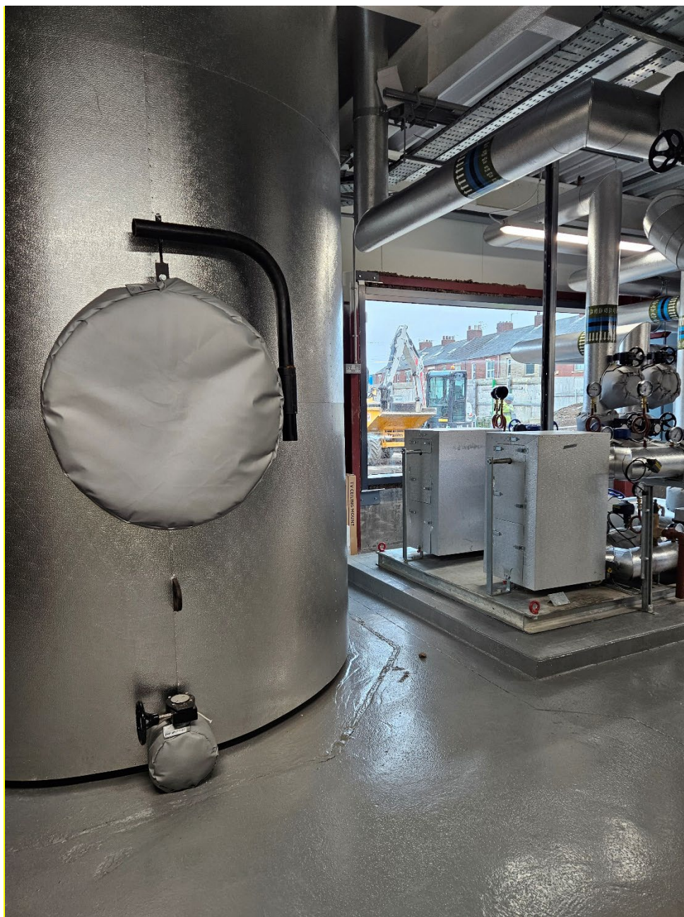
The thermal store and Durham Court heat exchangers are shown in the above image.
