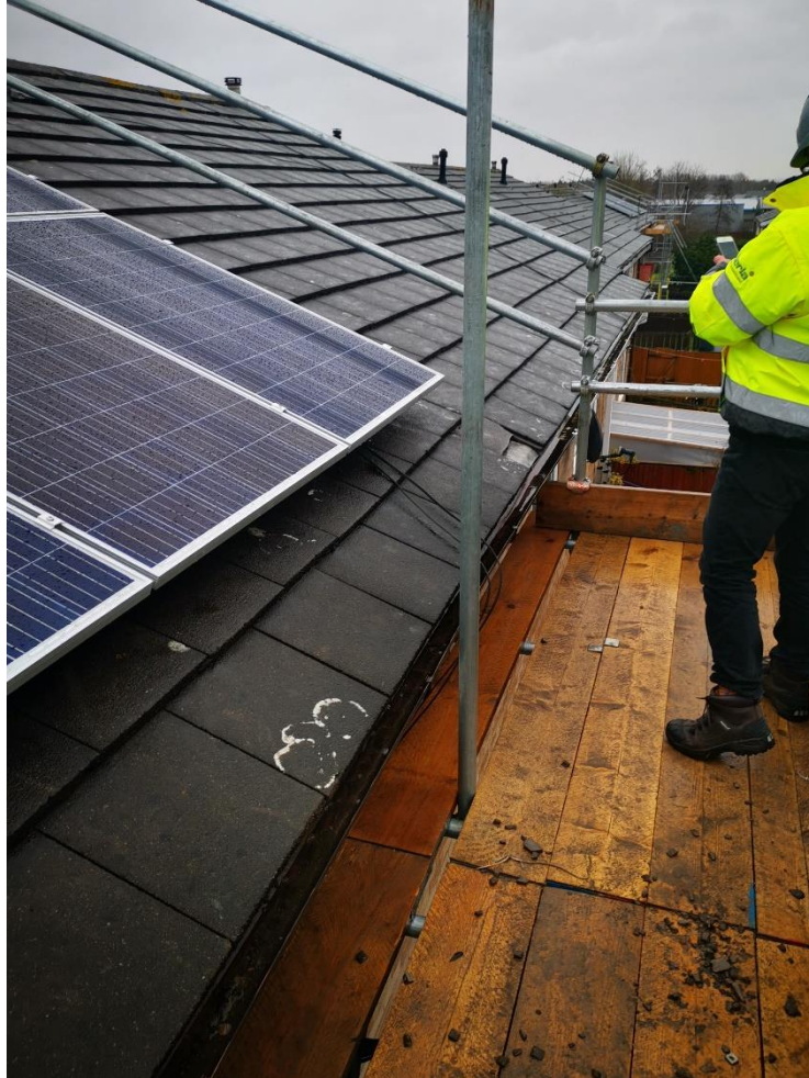
Installation of PV Panels in Ellesmere Port
