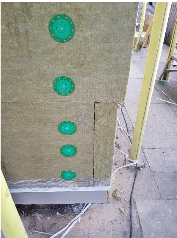
Typical Installation of EWI
