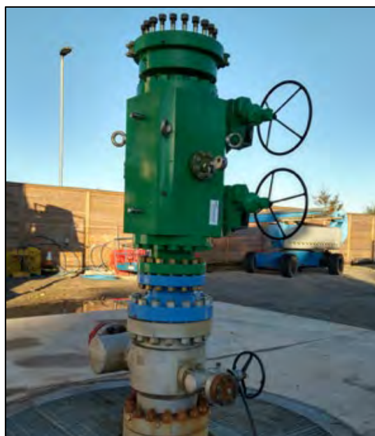
Hartmann master valve on UD-1 prior to testing
