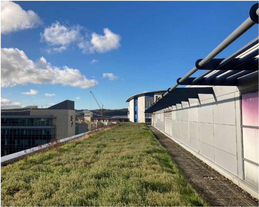
Image 11 – Existing Means of Escape
