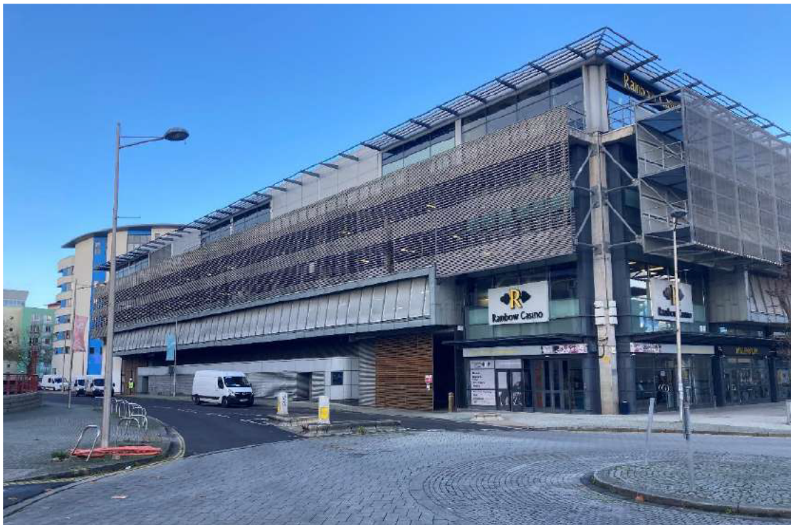
Image 2 – Rainbow Casino, Building 11 (viewed from Canons Way roundabout)
