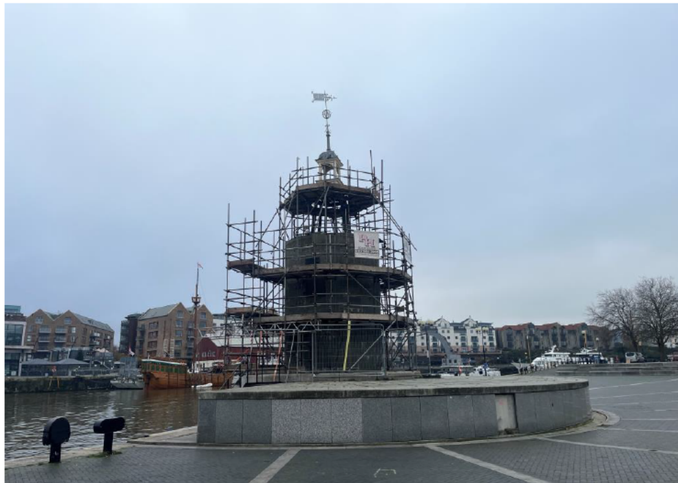
Figure 12: Grade II listed Crane Base
