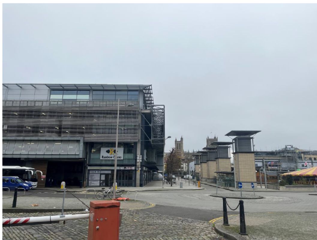
Figure 8: Example of view within the conservation area (looking north from Millennium Square where Bristol Cathedral can be seen
