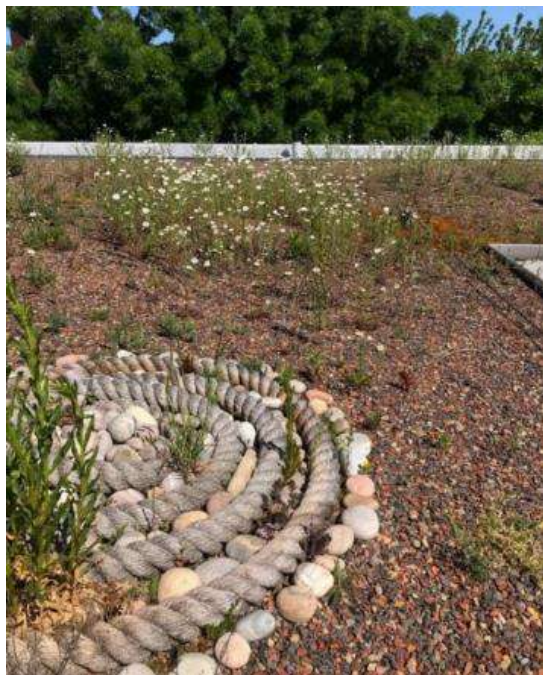
Plate 1.5 Rope coil on biodiverse roof
