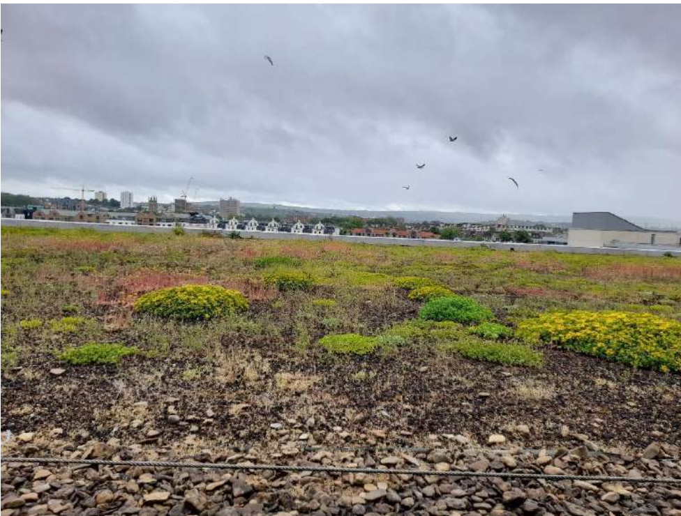
Plate 1.2 Existing sedum green roof
