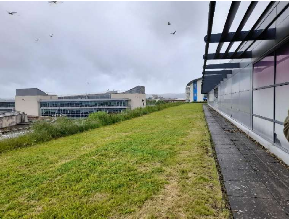
Plate 1.2 Existing sedum green roof
