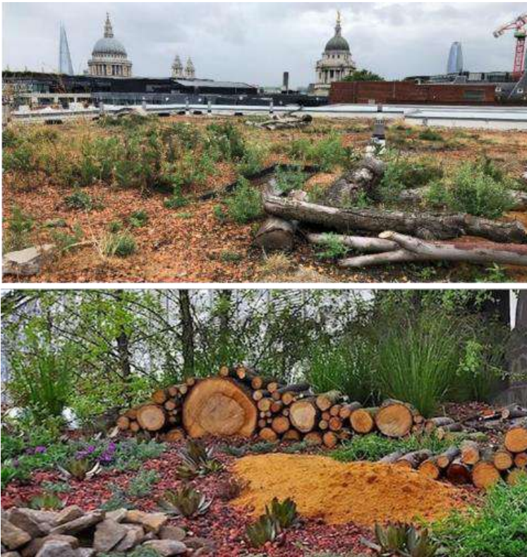
Plate 1.3 Examples of Log piles on biodiverse roofs
