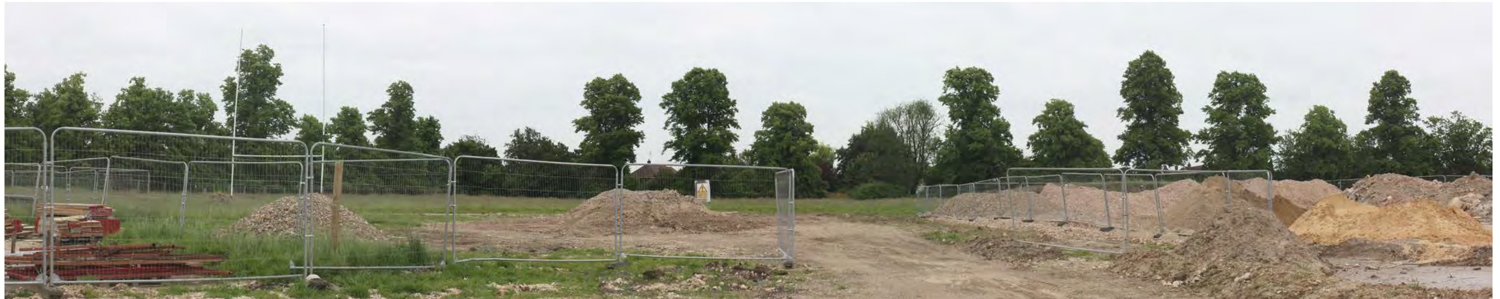
Contextual Photograph 5 View from south-eastern part of Site looking west
