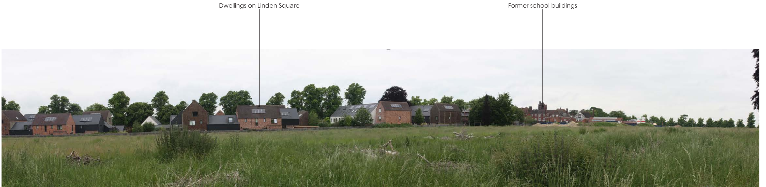
Contextual Photograph 7 View within Site to east of Pavilion Way looking north
