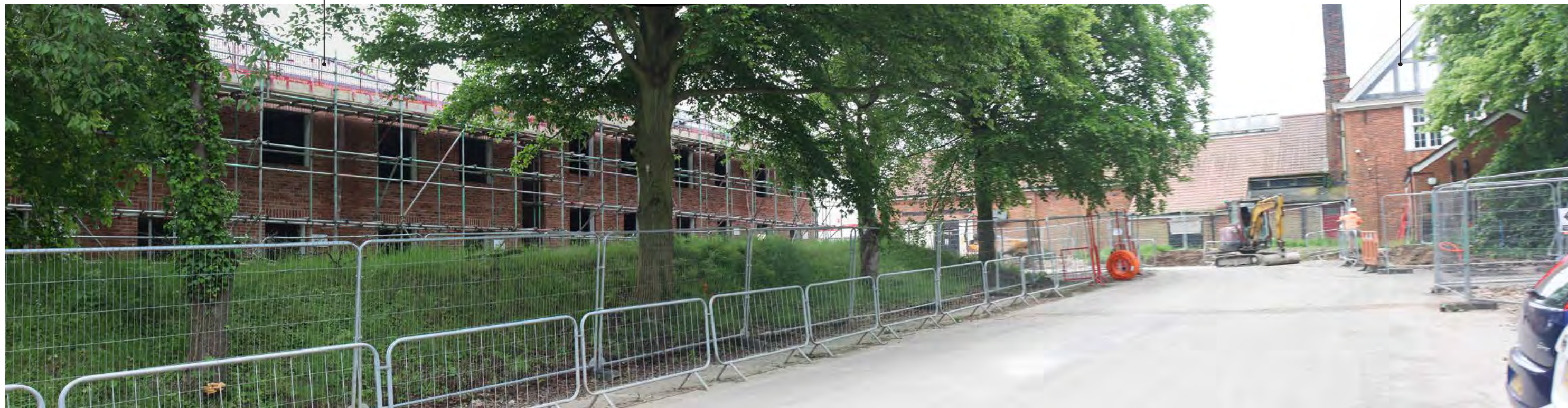
Photograph 9 View from northern end of entrance drive
