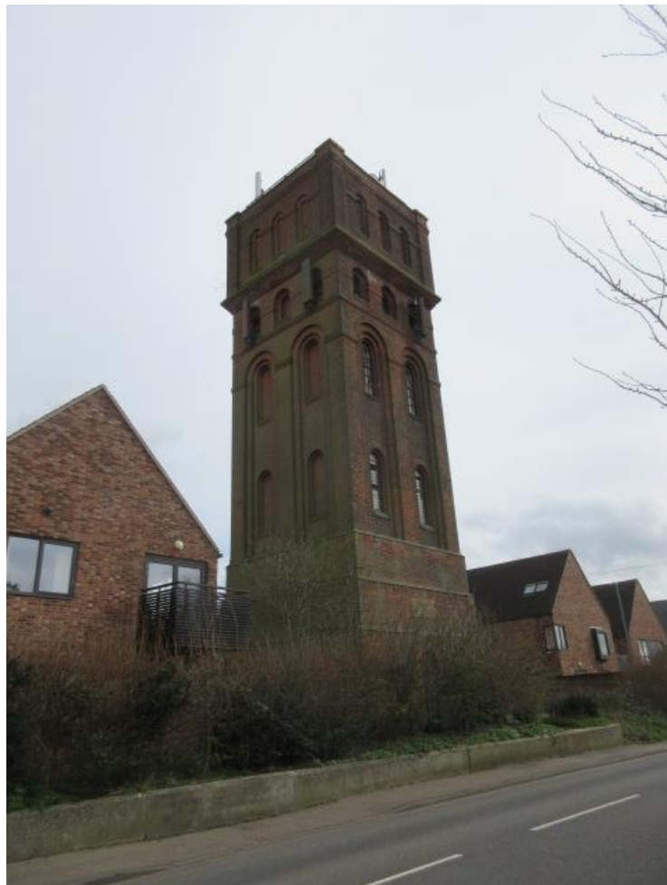
Plate 4: Listed water tower, looking south east
