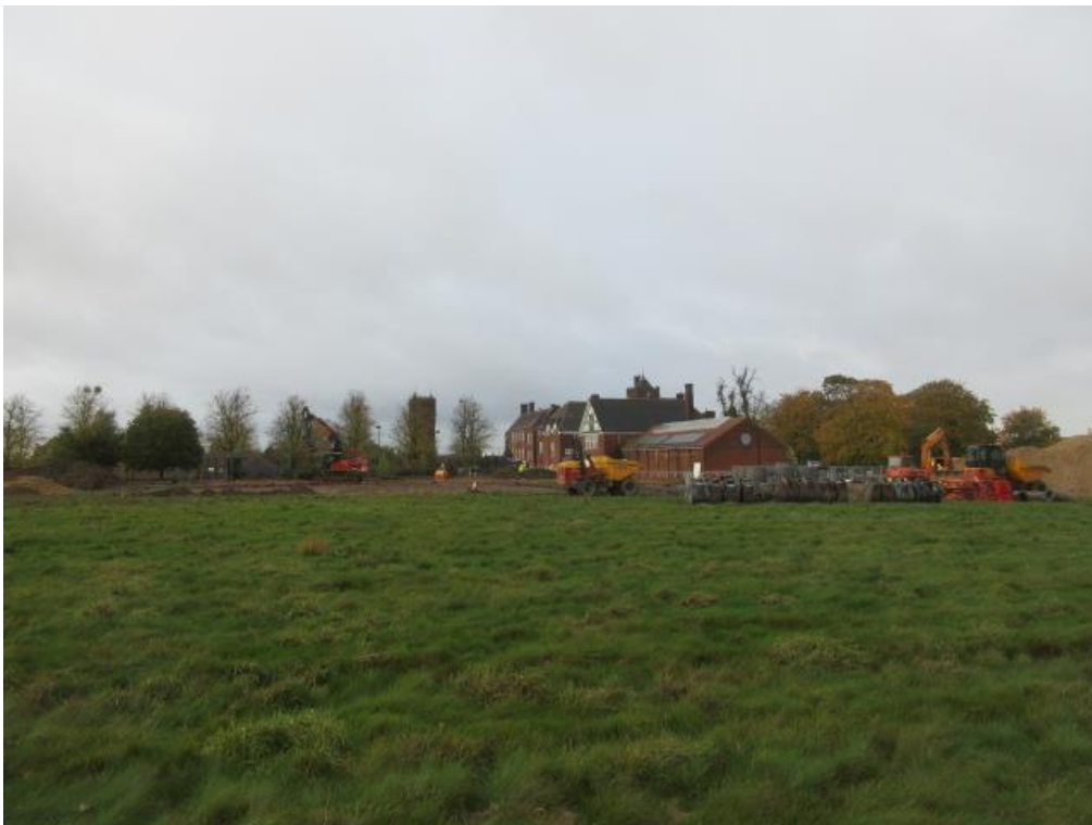
Plate 12: Main school buildings from site, looking north west
