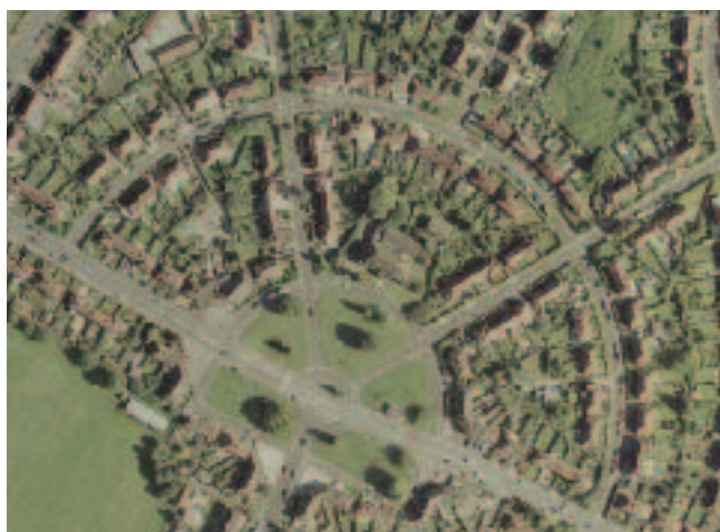
Some houses form part of a formal layout such as the above 'garden city suburb' at Seamills
