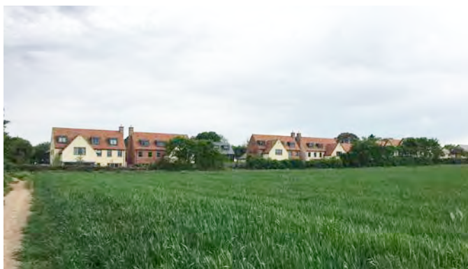
▲ Modern dormer windows create character at Thorpe Lea Close in Great Chesterford.
