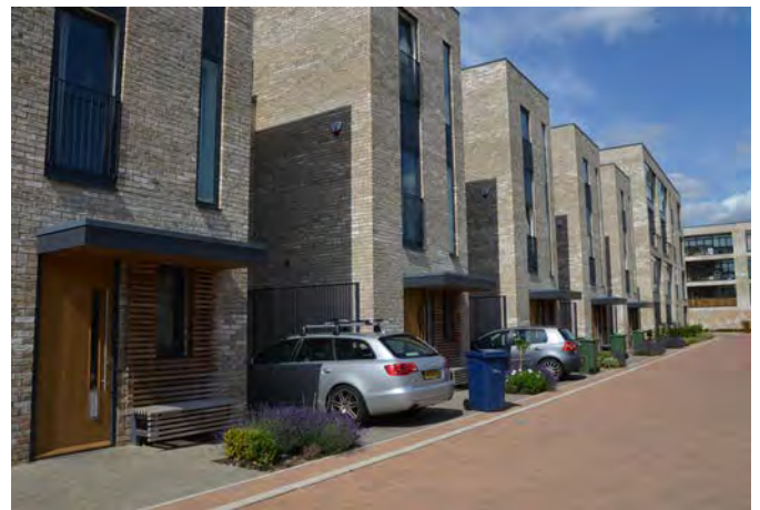
▲ Visual impact of parking space projecting beyond the building line is reduced with planting and strong frontage.
