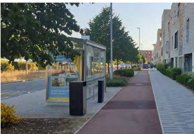
▲ Bus stops provided with suitable space to safely embark / disembark, whilst safely separated from the adjacent cycleway.
