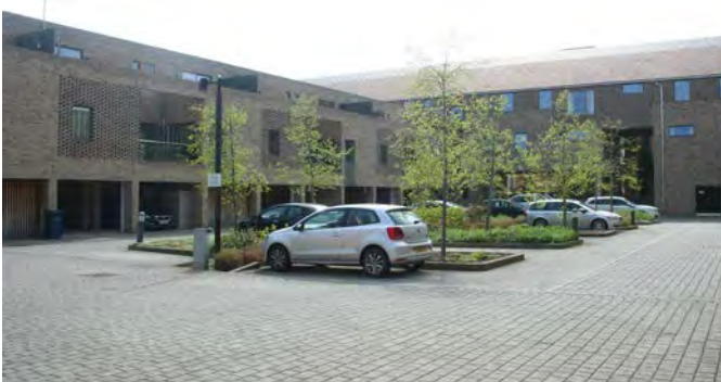
▲ Well-designed parking court with permeable paving and space for servicing and utilities.
