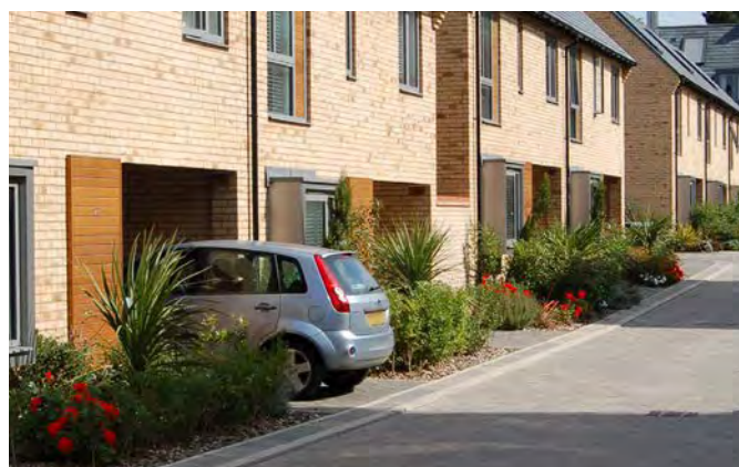
▲ On-plot parking is integrated into the street scene with soft landscaping to create an attractive streetscape.
