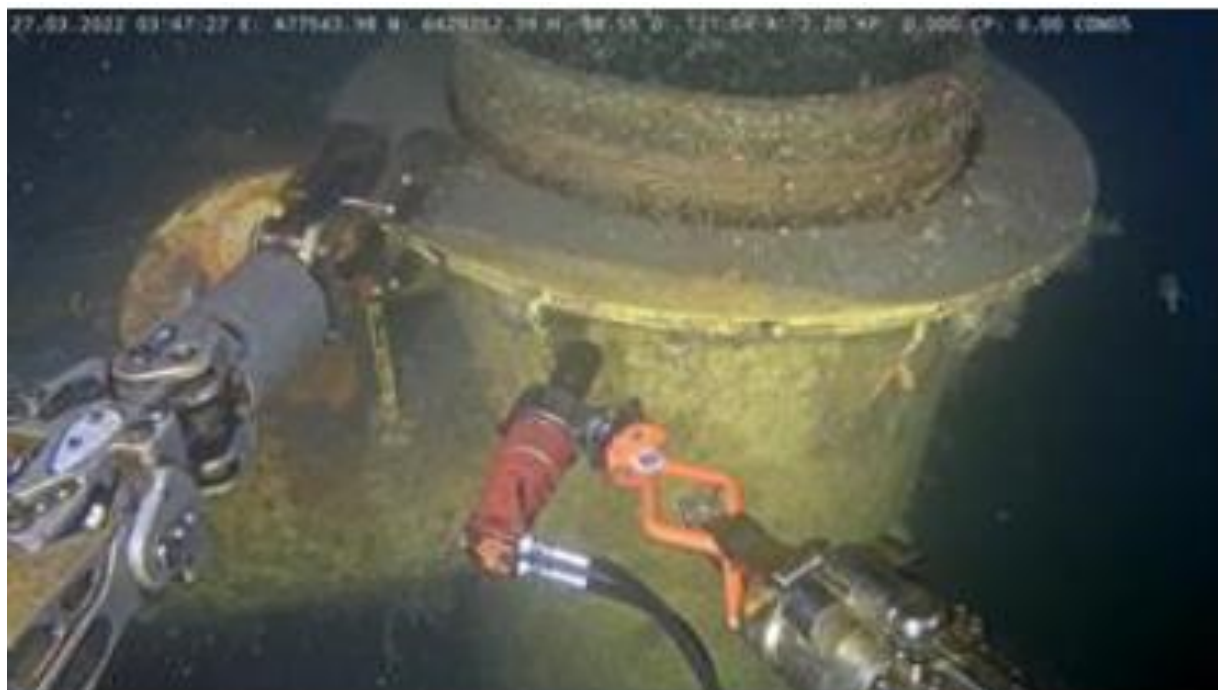
Figure 8.4: Removing continuity bolt during SSIV recovery
