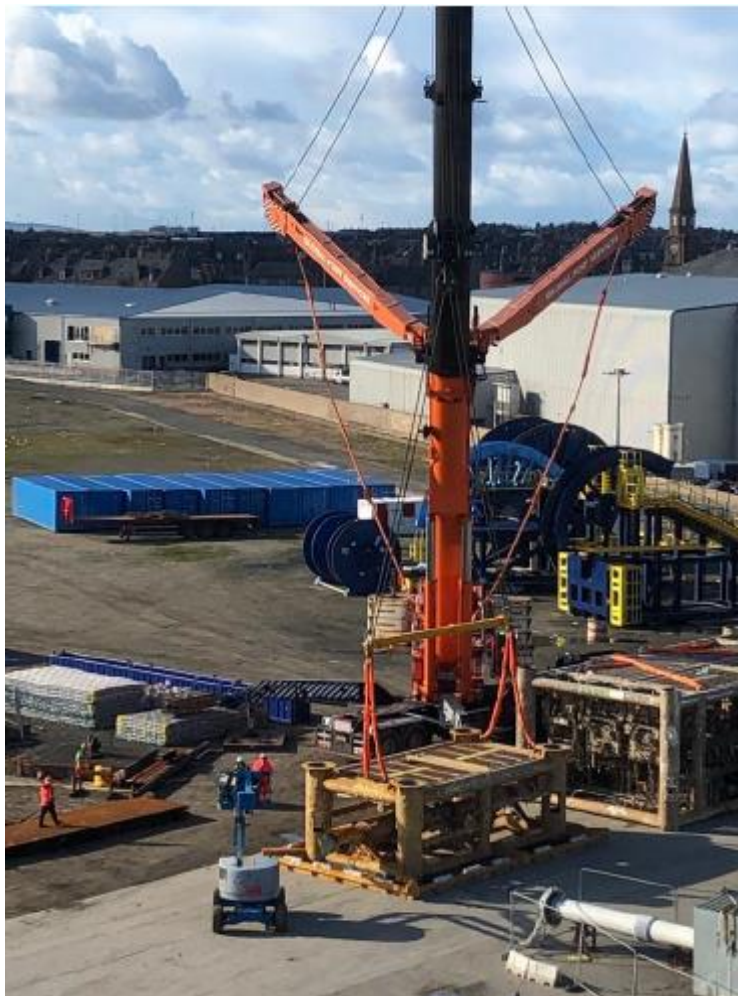
Figure 8.5: Goldeneye SSIV offload at quay
