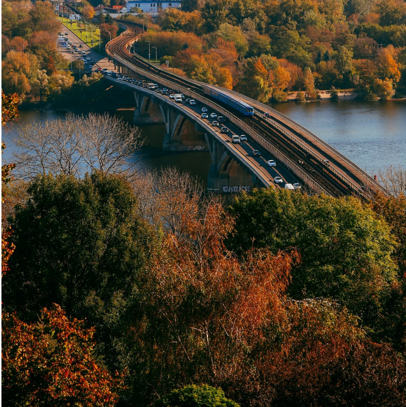
A road and rail bridge crossing a river surrounded by trees.
