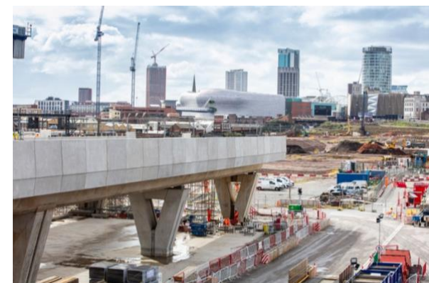
Construction progress at Curzon Street viaduct, Birmingham.
