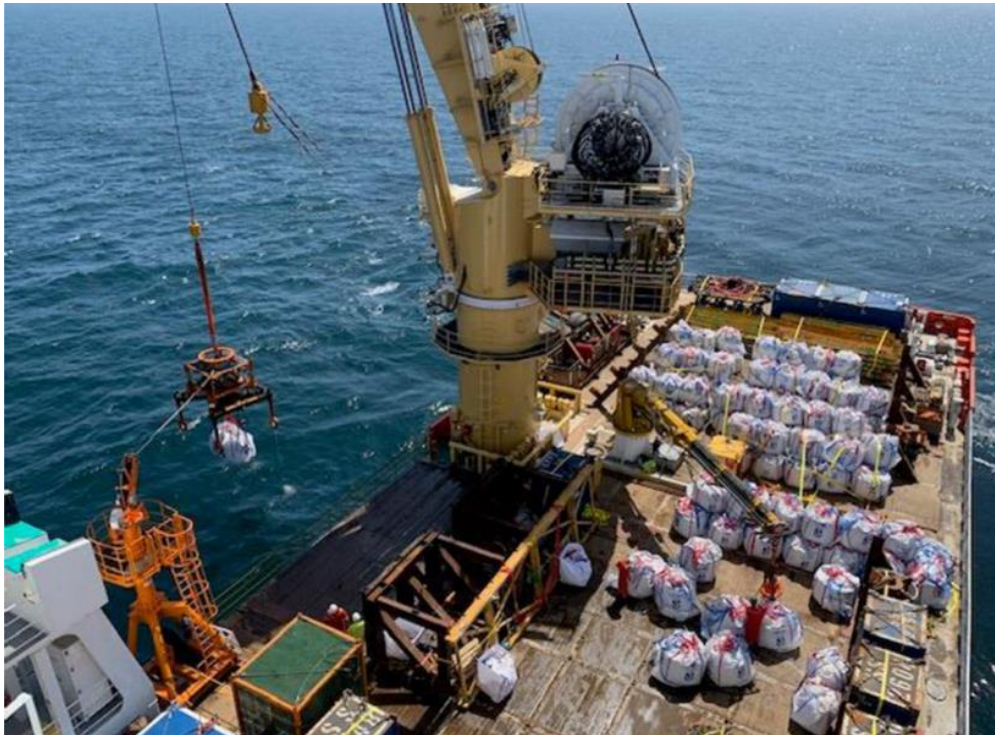
Figure 2-4. Schooner & Ketch Pipeline Decommissioning (June 2023)
