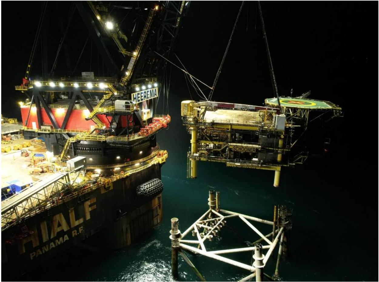
Figure 2-2. Schooner Topside Removal (May 2023)
