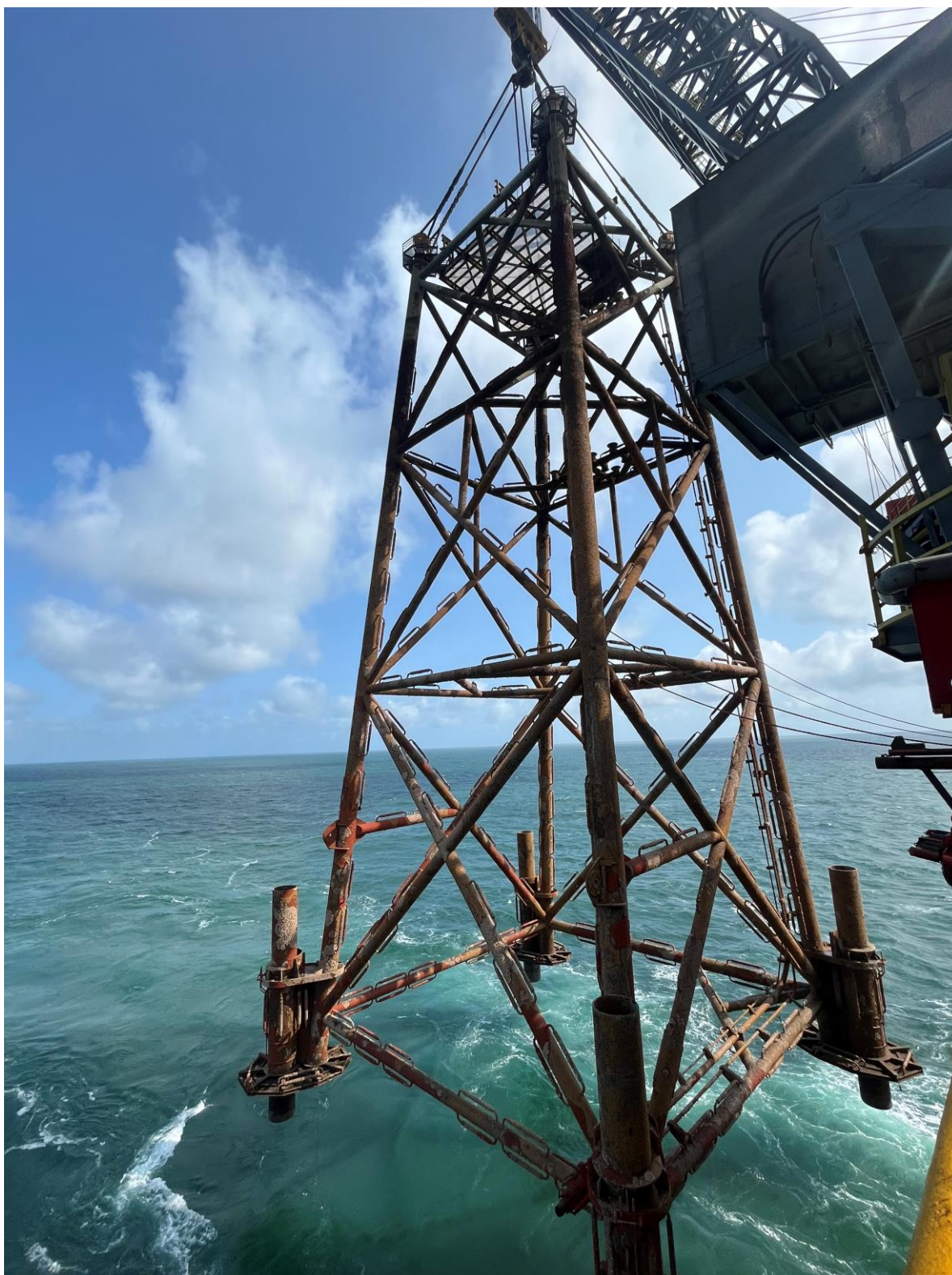
Figure 2-3. Schooner Jacket Removal (May 2023)
