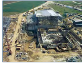
Construction progress of JET in the 80s
