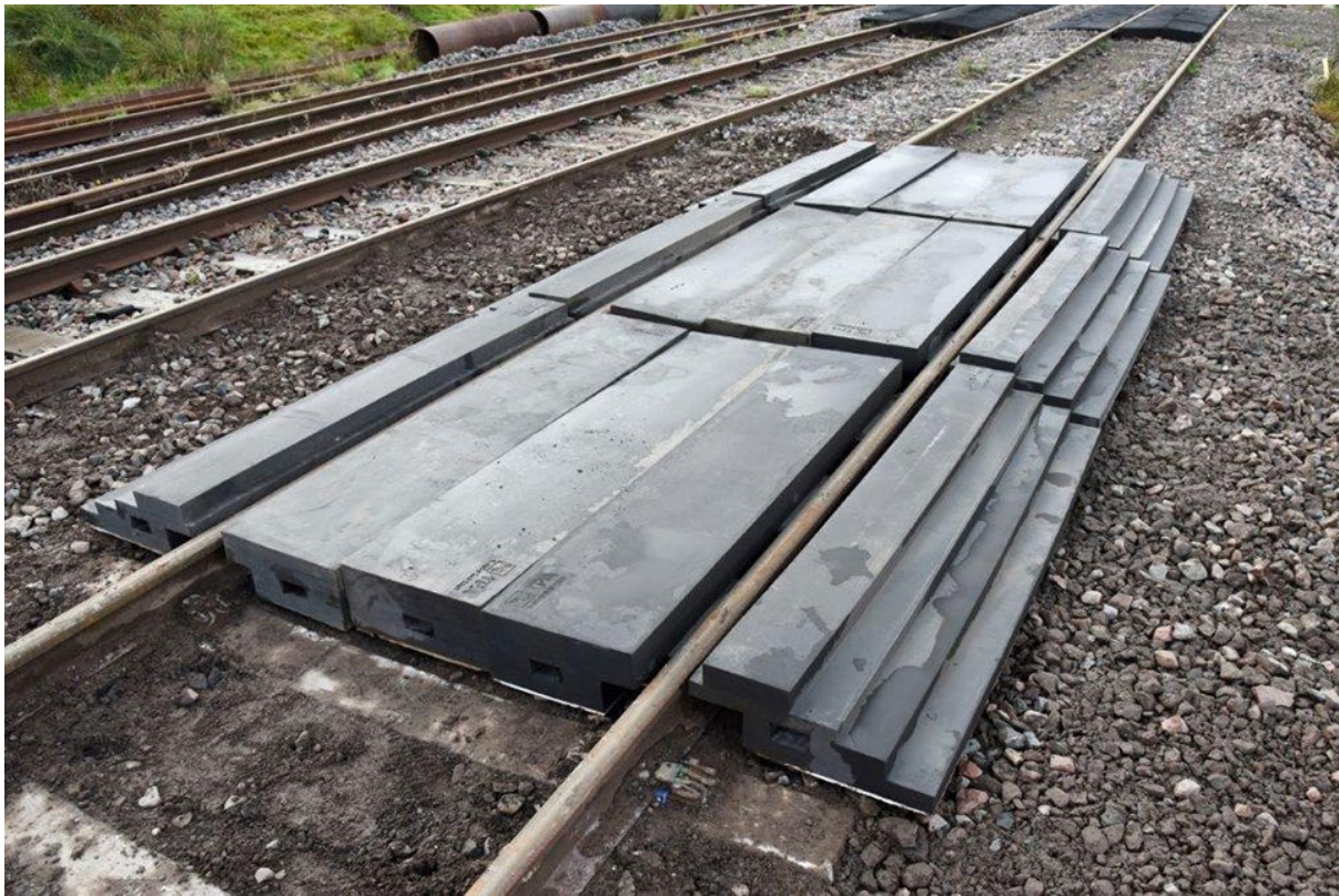
High density foam temporary RRAP kit installation demonstration (courtesy of VP plc).
