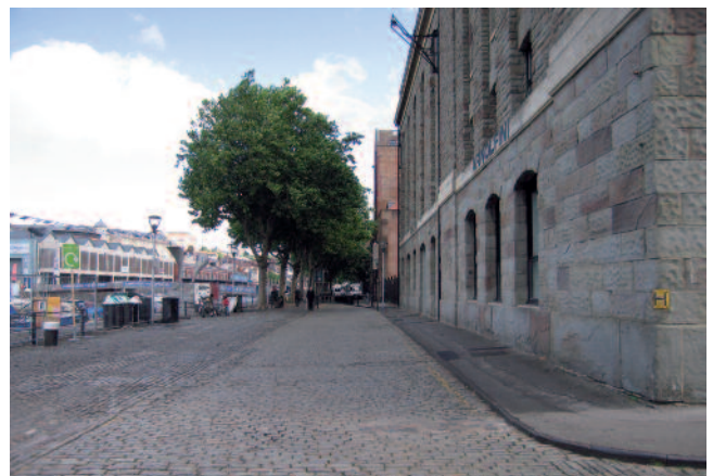
Figure 18: Narrow Quay looking north
