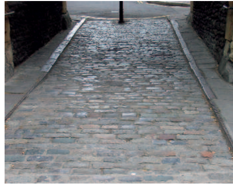
Figure 32: Traditional street surface at St John's on the Wall
