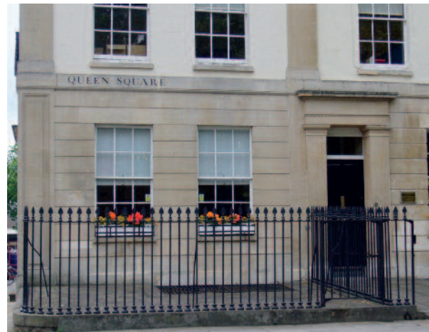
Figure 33: Railings with spear-point finials
