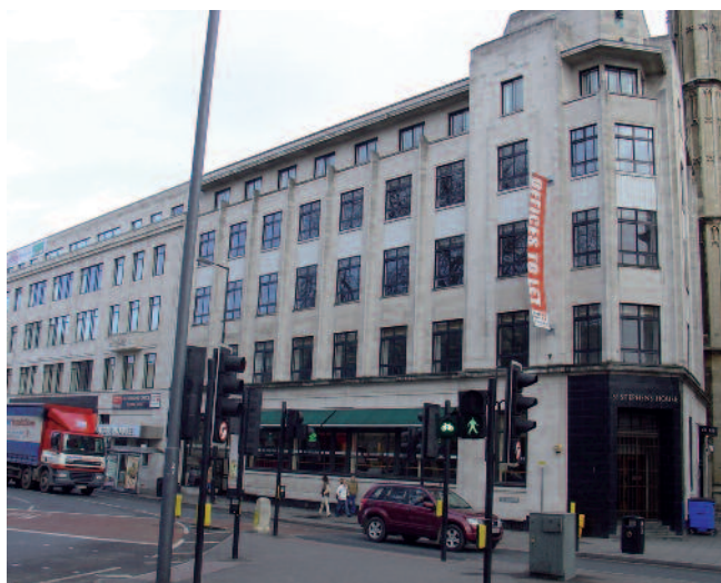
Figure 36: St Stephen's House
