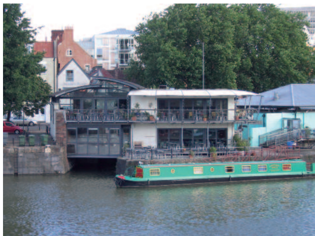
Figure 35: River Station Restaurant
