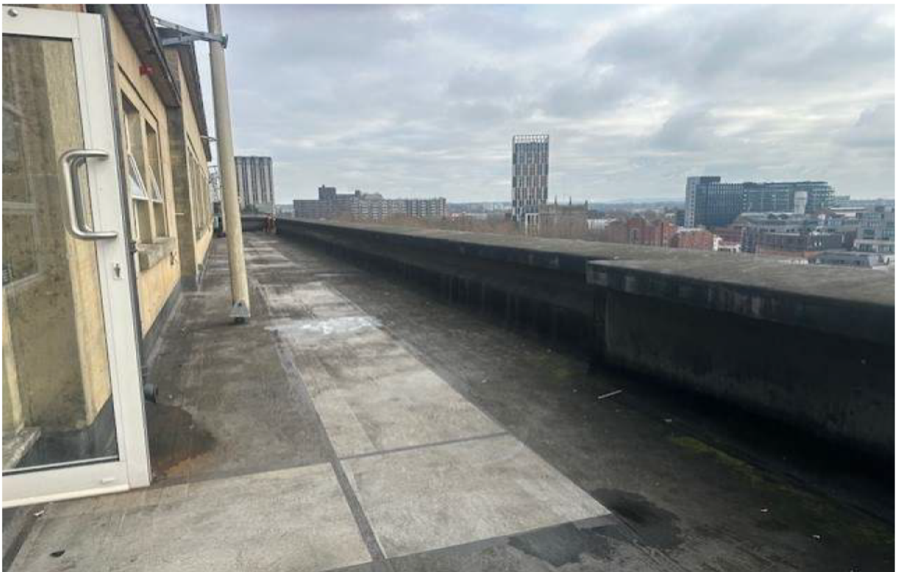
Photograph 2: Balcony area looking east
