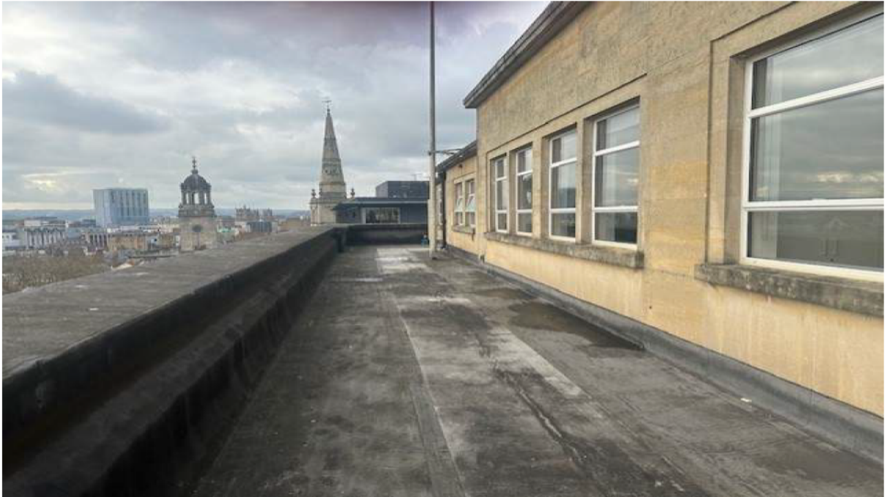
Photograph 1: Balcony area looking west
