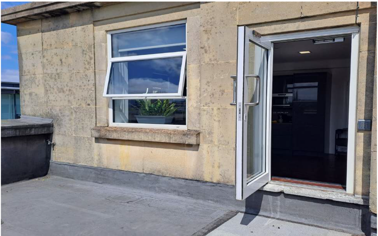
Photograph 4: Access door to balcony area from kitchen
