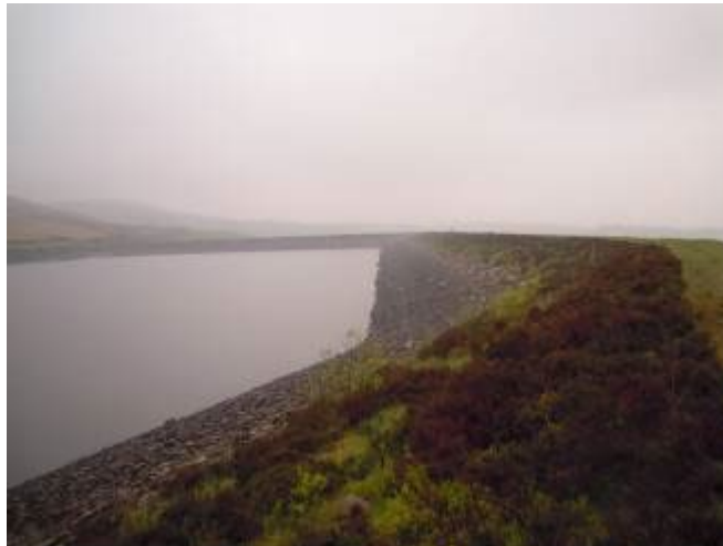
Figure C4.1: Sunnyhurst Hey Reservoir (source: Dr Andrew Hughes, Dams and Reservoirs Ltd)
