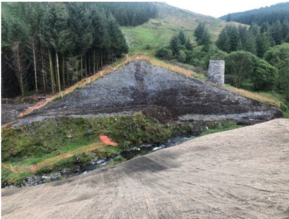
Photograph 1: Cut section through a discontinued dam showing vertical peat core (source: Dr Andrew Hughes, Dams and Reservoirs Ltd)
