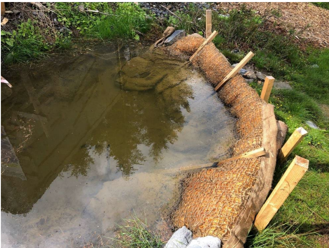
Photograph 6: Example of a silt trap barrier across a watercourse (source: Dr Andrew Hughes, Dams and Reservoirs Ltd)
