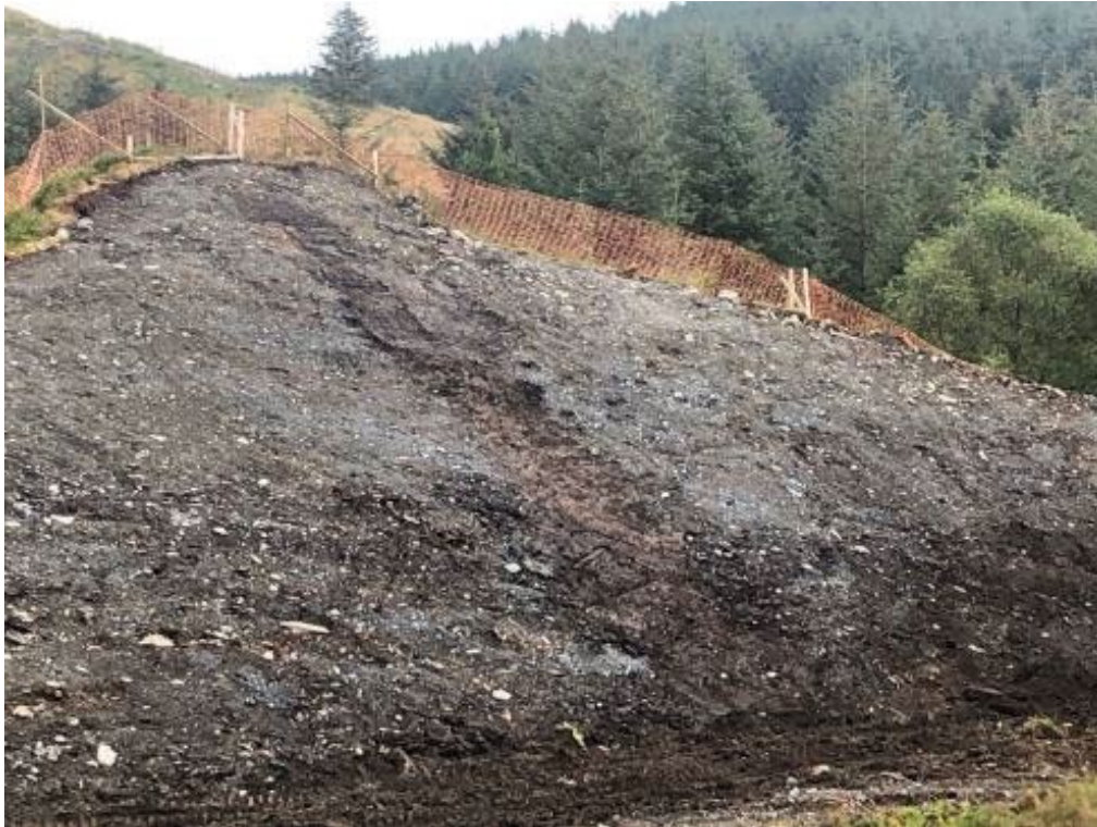
Photograph 2: Cut section through a discontinued dam showing peat core (source: Dr Andrew Hughes, Dams and Reservoirs Ltd)
