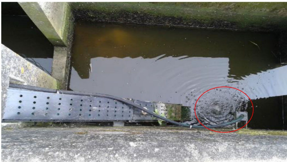
Figure 5: Eel pass at Judas Gap after modification by adding a flow splitter to provide attraction flow at the base of the pass (red circle) (source: Adam Piper)
