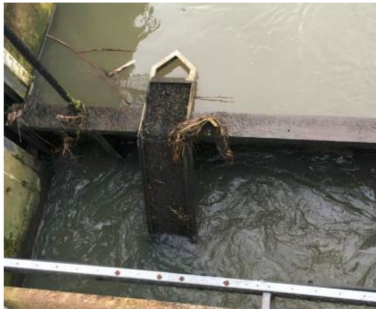
Figure 17. Hook-over gravity fed eel pass with debris deflector at the upstream end, deployed on Bargate sluice in Lincolnshire (source: Hugh Bunker/James Hooker)
