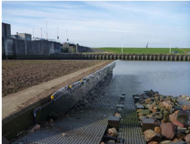
Figure 22: Elver pass at Nieuwe Statenzijl, Netherlands with multiple plunging flow outlets to enhance attraction to the downstream end of the pass (source: Peter Paul Schollema)
