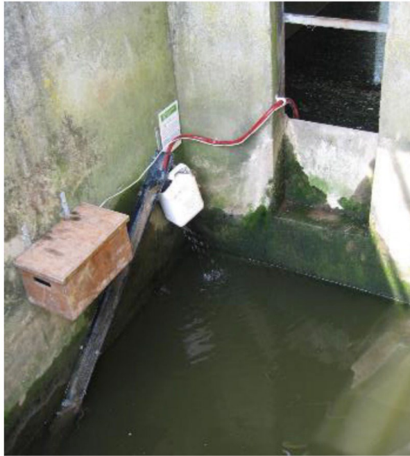
Figure 4: Simple trough-type elver pass with conveyance flow supplied by a bilge pump, powered by 12V leisure battery housed in wooden box fixed to the wall above the pass (source: Dan Hayter)
