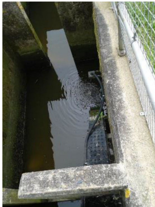
Figure 21: An eel pass at Judas Gap after modification – flow splitter added to deliver attraction flow to the base of the pass (source: Adam Piper)
