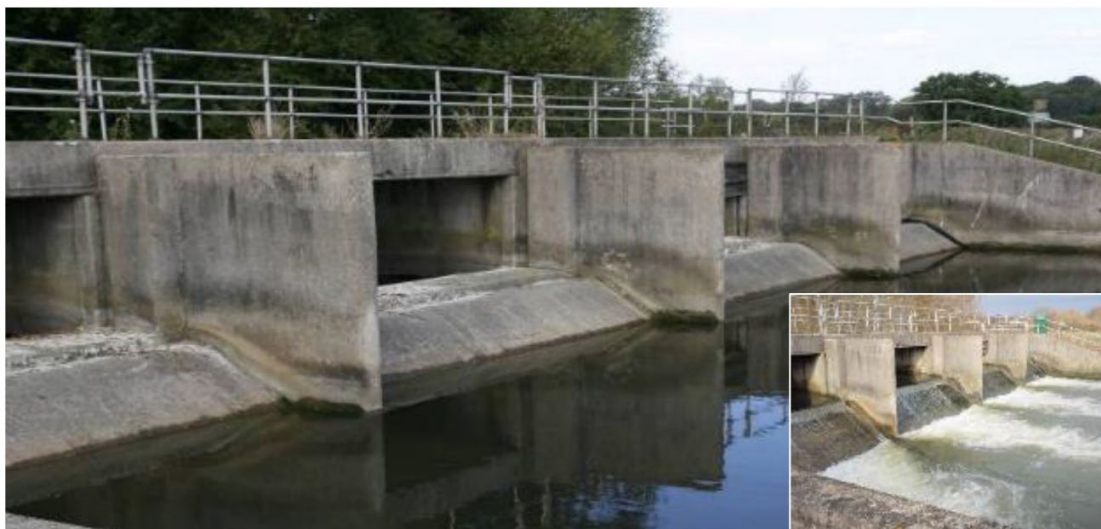
Figure 3: Judas gap weir on the River Stour in Essex when not spilling - and inset image shows during high winter flows (source: Adam Piper)
