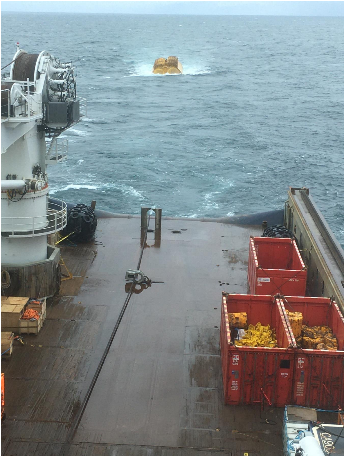
Figure 9.5.1: Mid-Water Arch viewed from back of AHV
