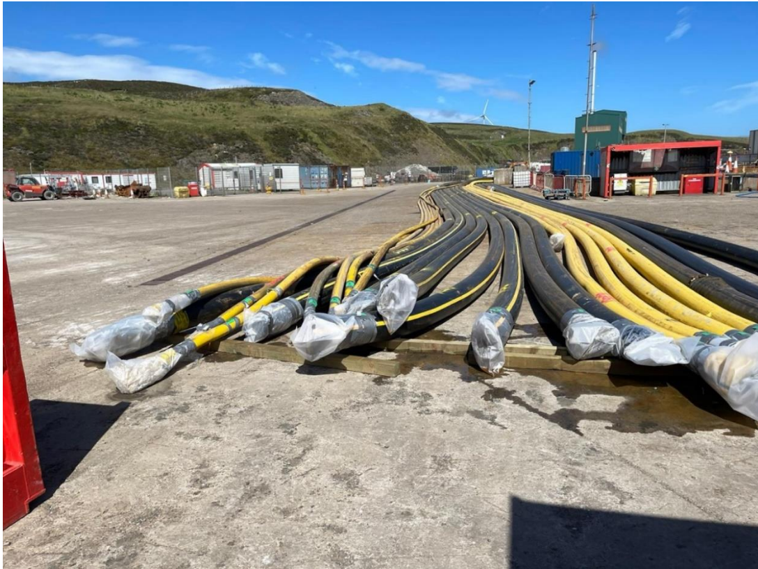
Figure 9.4.3: Flexible risers and umbilical risers in Lerwick
