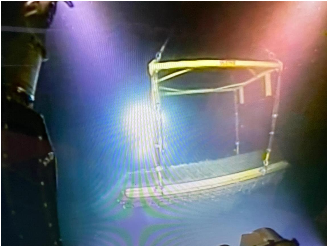
Figure 9.6.1: Concrete mattresses being recovered using a "Speedloader"
