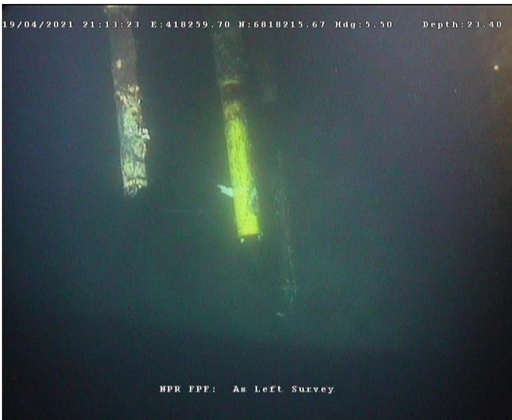
Figure 9.3.2: Cut flexible riser and umbilical
