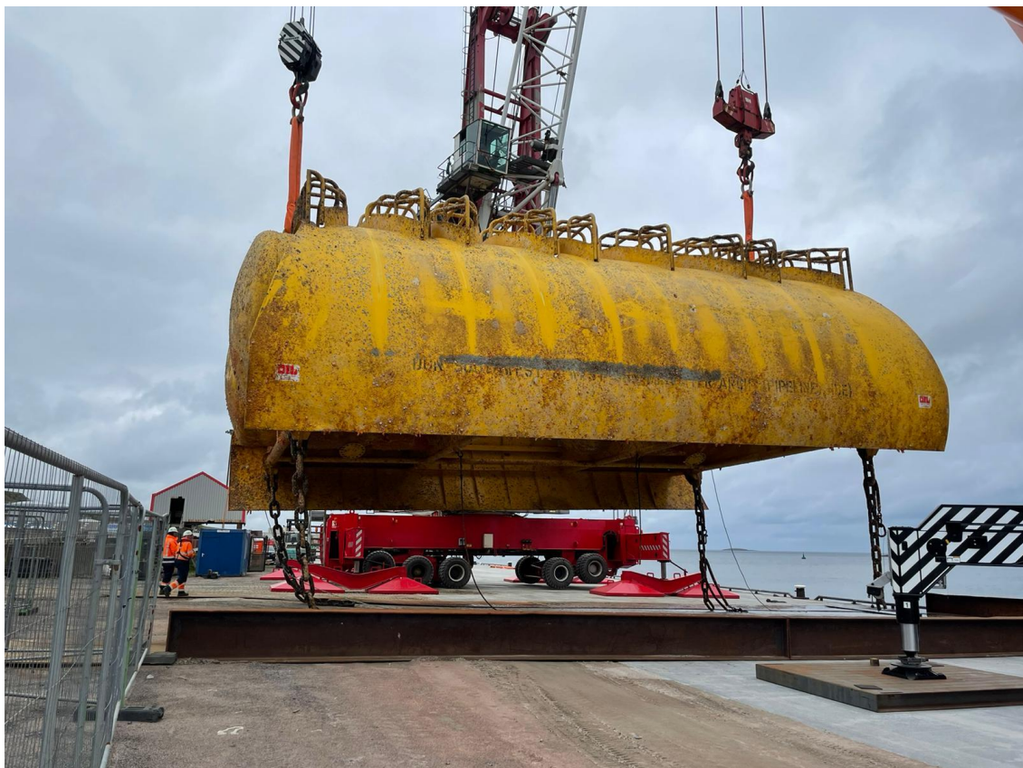
Figure 9.5.4: Mid-Water Arch lifted onto quayside
